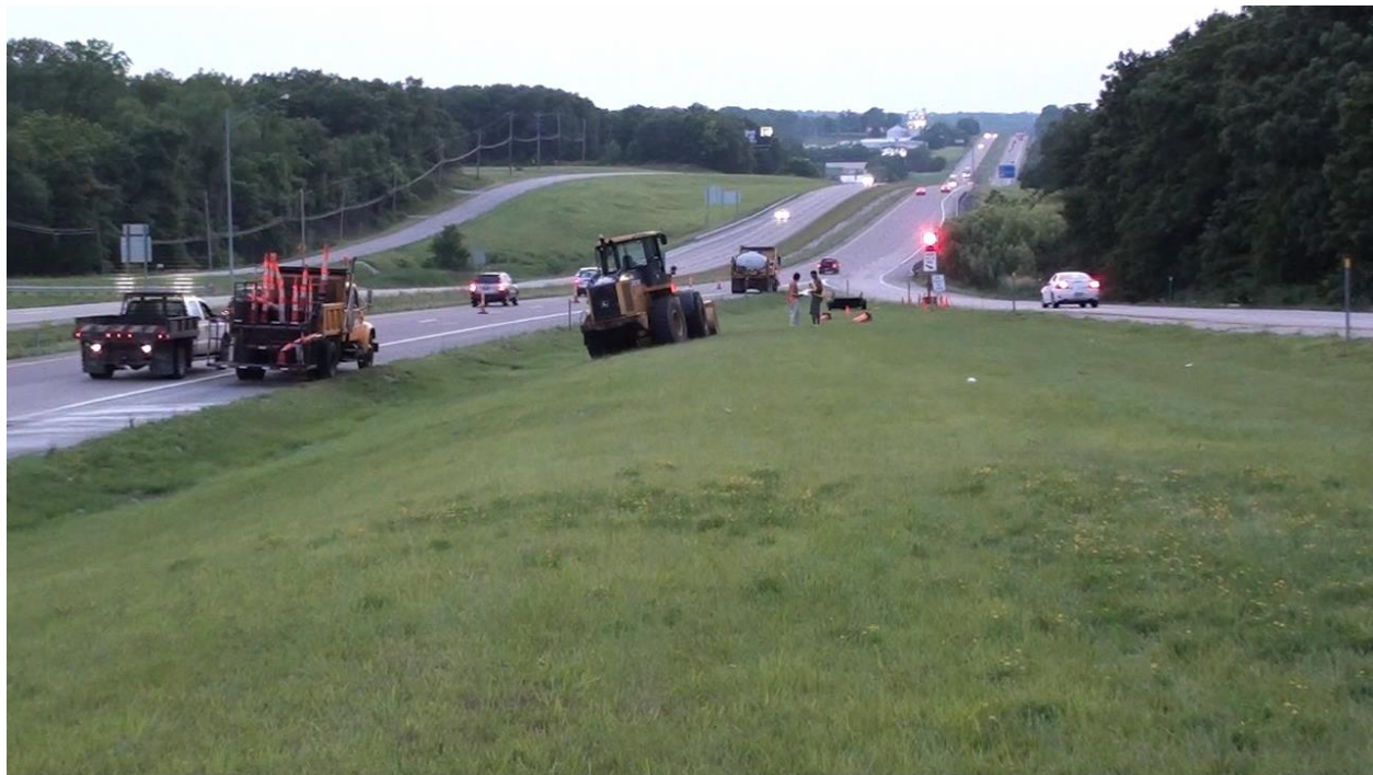
Figure 2.5 I-70 WB at mile marker 131, two-head signal.
