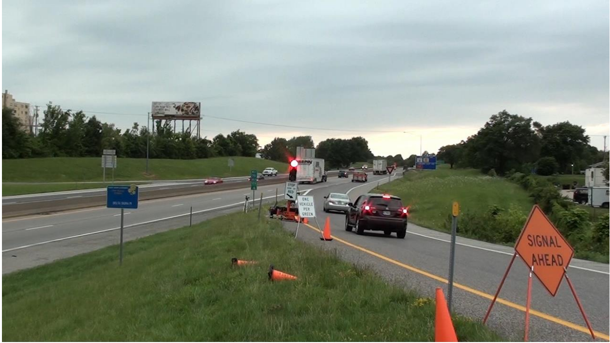
Figure 2.8 I-70 WB at mile marker 126.6.
