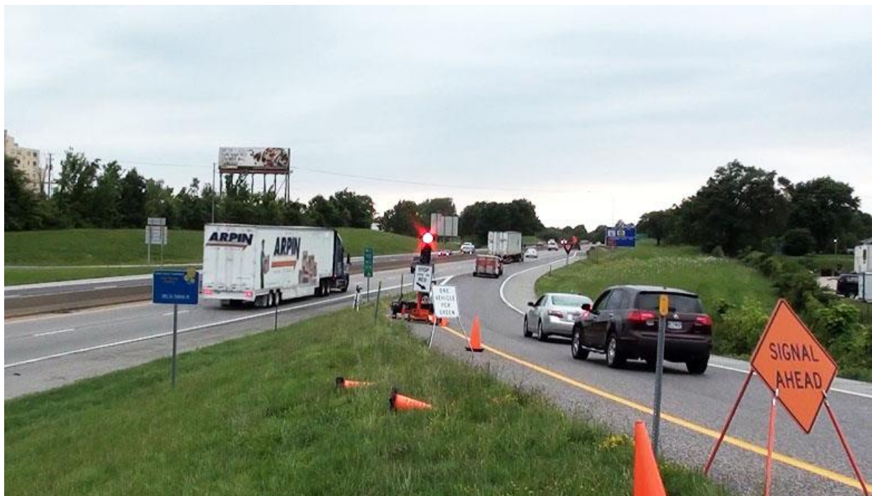
Figure 2.2 Ramp metering in operation.
