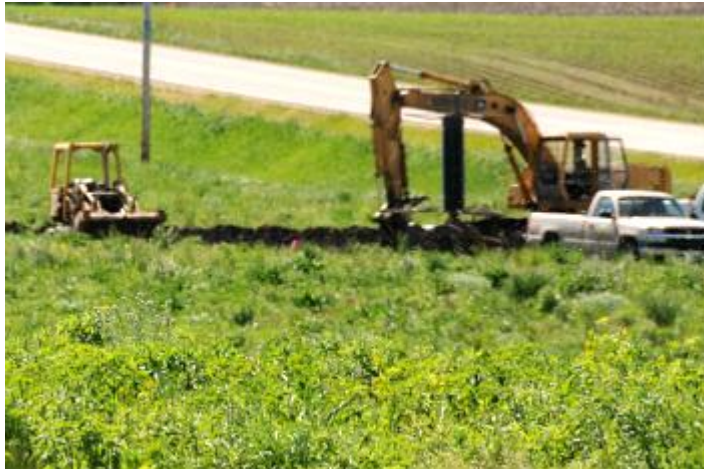
Drainage Tile Installation
