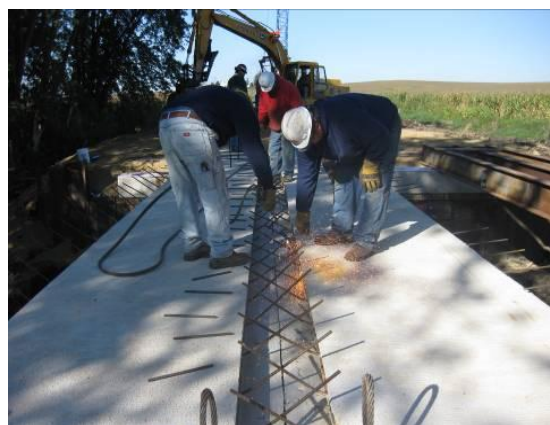
Figure 5-31. Finishing of bridge deck joints
