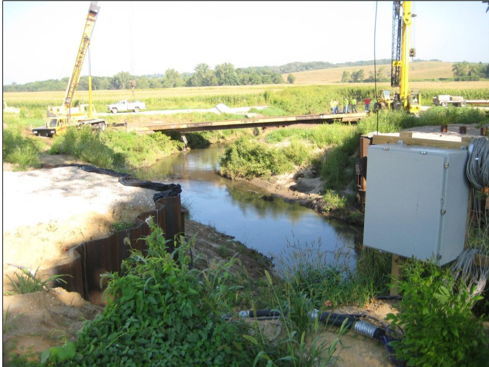
Figure 5-131. Lifting temporary deck into place (August 13, 2010)
