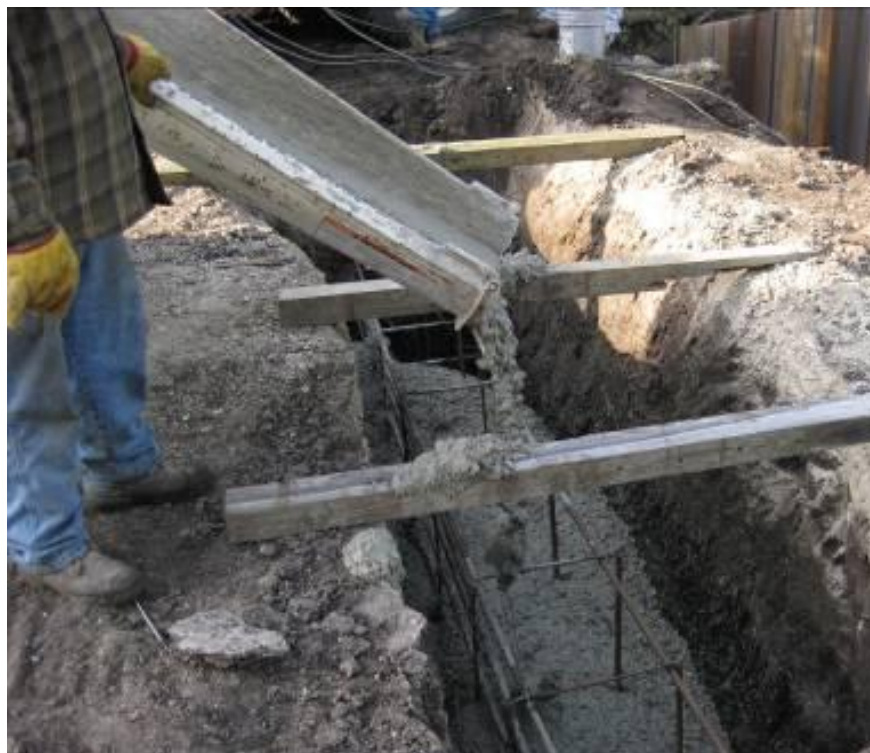
Figure 5-19. Reinforced concrete deadman placement behind east abutment
