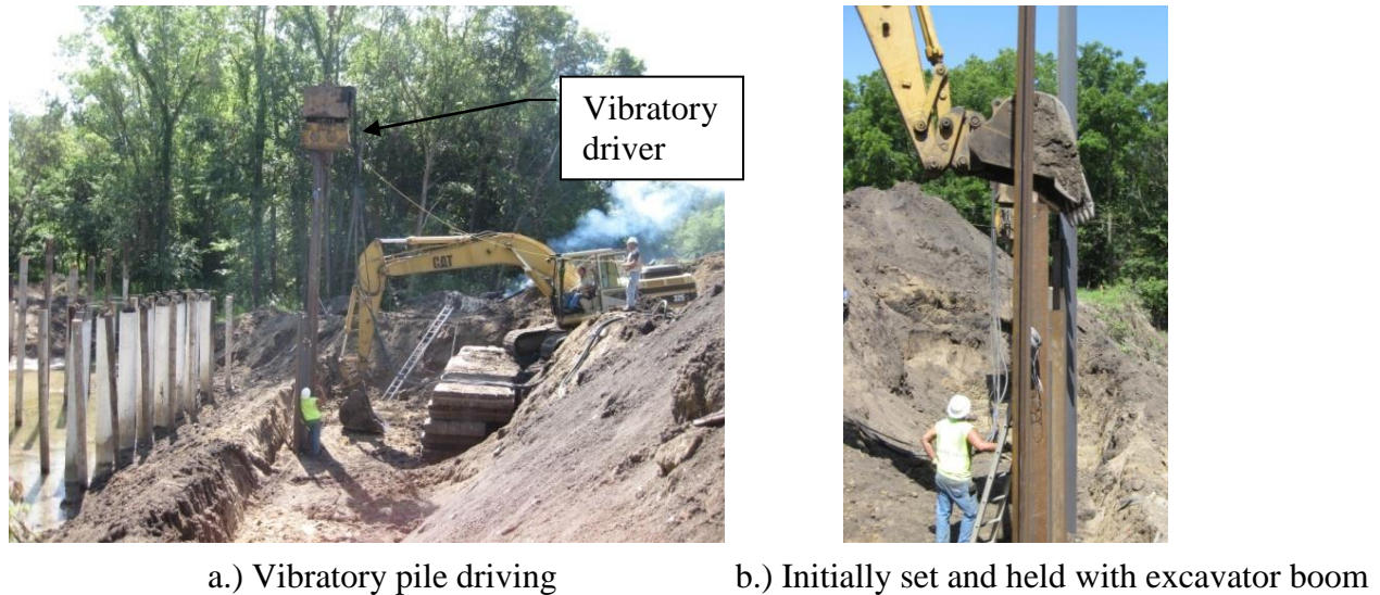
Figure 5-66. Placement of sheet pile sections
