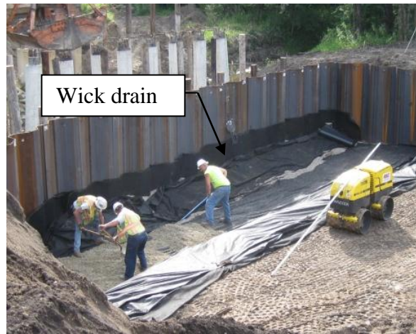
a.) Engineering fabric placement
