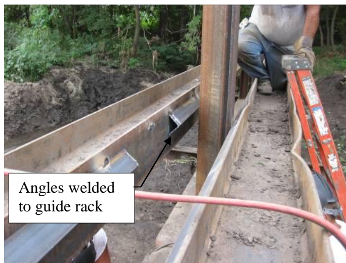
a.) Guide rack with angles attached
