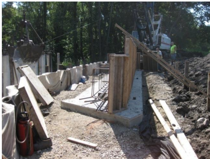
Figure 5-83. Reinforced concrete spread footing on west abutment
