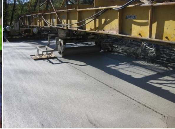
b.) Screeded to form 1% crown
