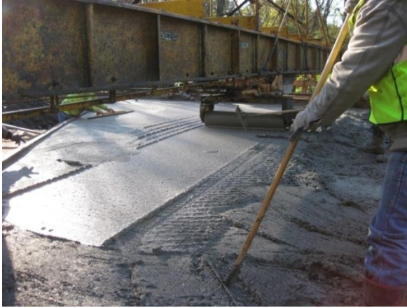
a.) Unfinished concrete after placement
