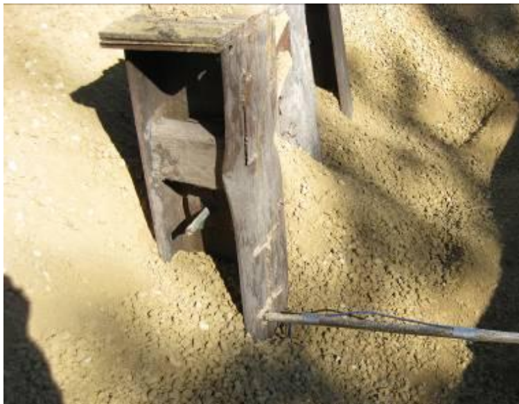
Figure 5-21. Tie rod to H-pile connection
