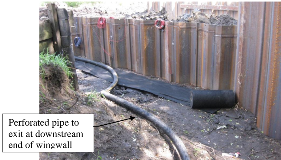
Figure 5-18. Drain tile installation on backfill side of west abutment in BHC, Iowa
