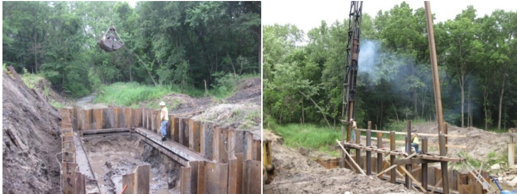
a.) Cofferdam placement and excavation b.) Placement and driving of battered piles
