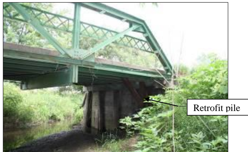
Figure 5-2. Previous bridge structure at demonstration project site in BHC, Iowa with retrofit pile
