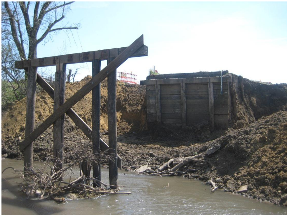
Figure 5-128. Partial demolition of existing bridge (April 14, 2010)
