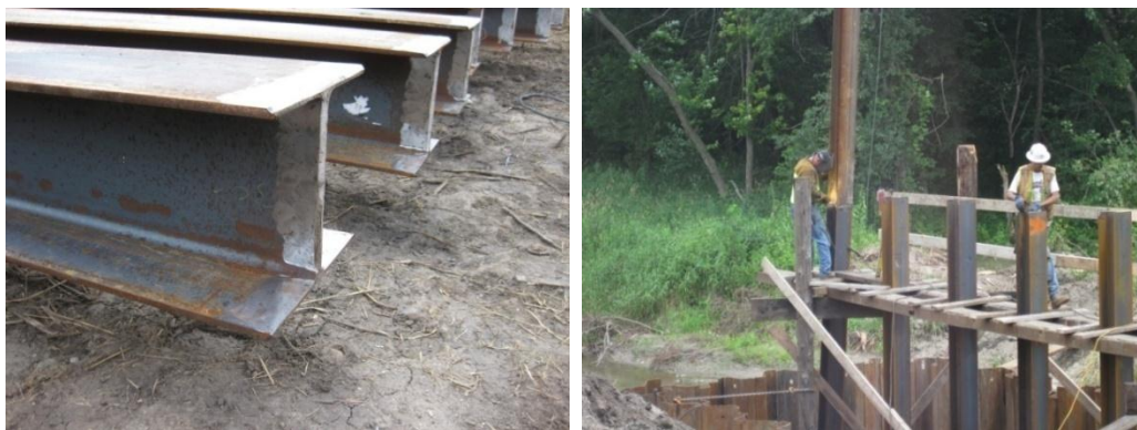
a.) Preparation of piles for welding b.) Welding two 40 ft sections together
