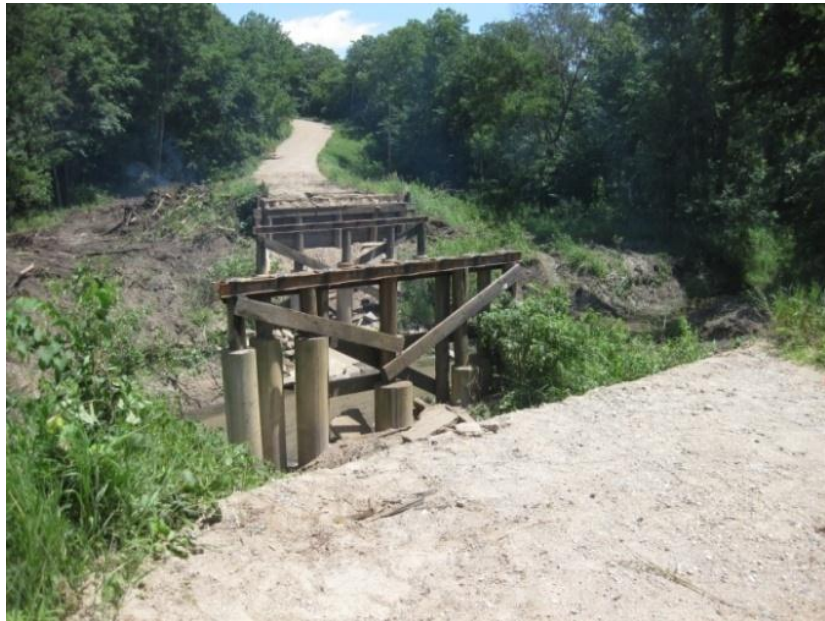
b.) Superstructure removed
