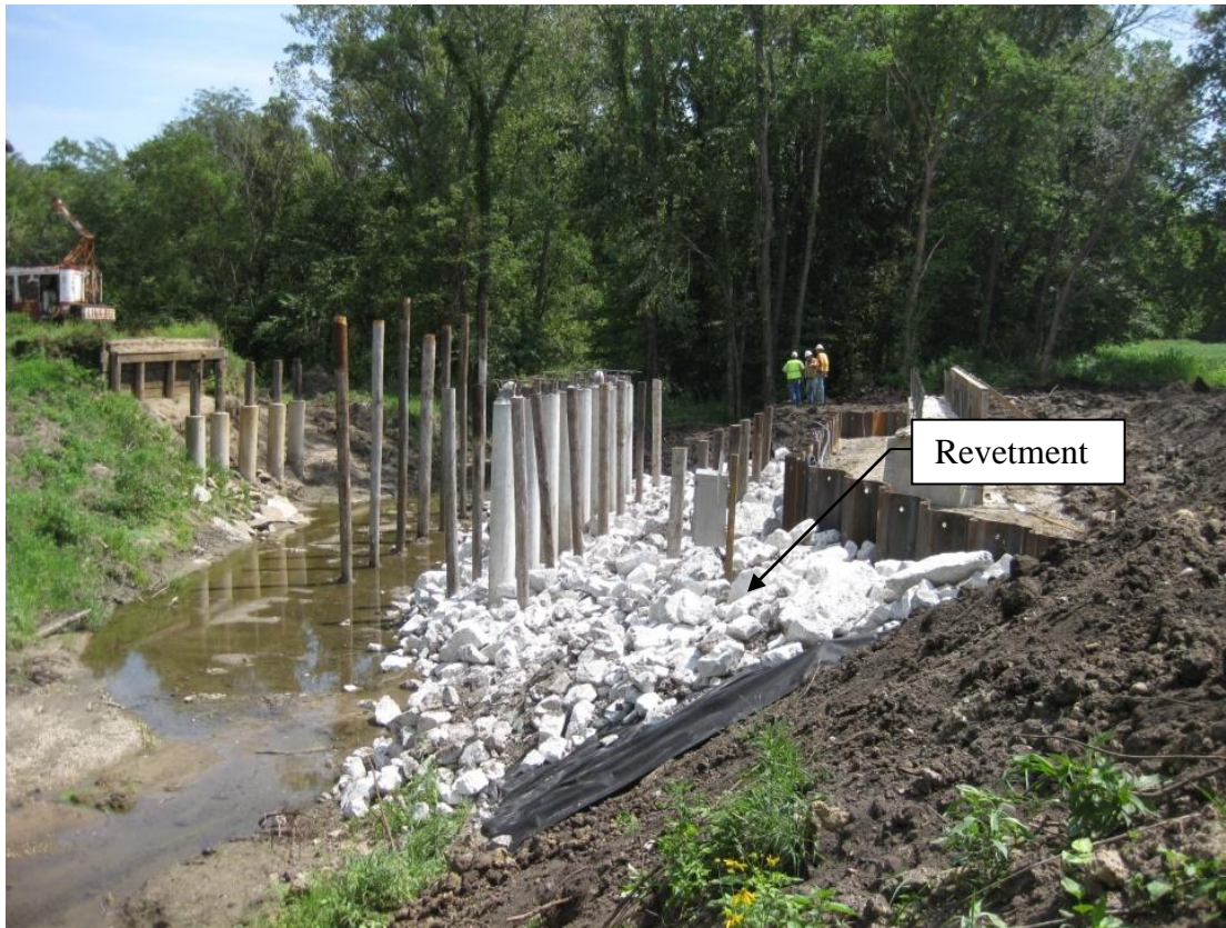
Figure 5-86. Finished west abutment and pier
