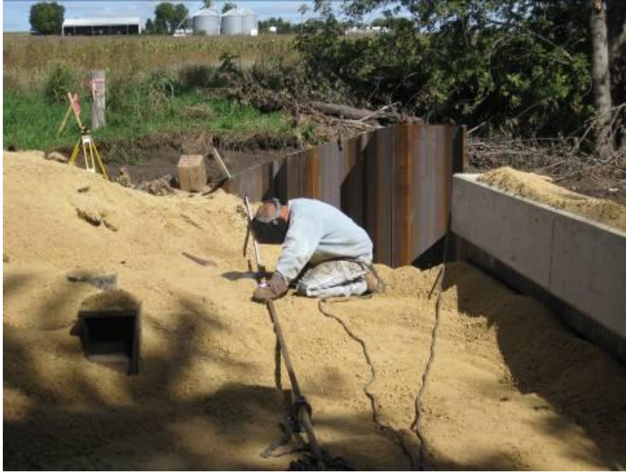
Figure 5-20. Installation of wingwall tie
