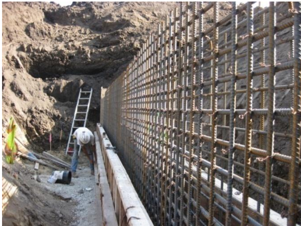
b.) Reinforcement and formwork being placed
