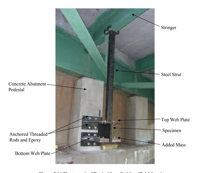
Figure 3.14 Photograph of Typical Installed Sacrificial Specimen
