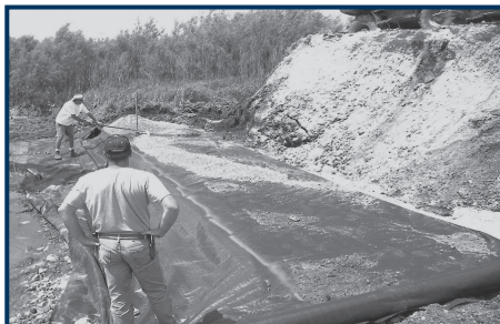
Starting with two layers as a curtain wall
