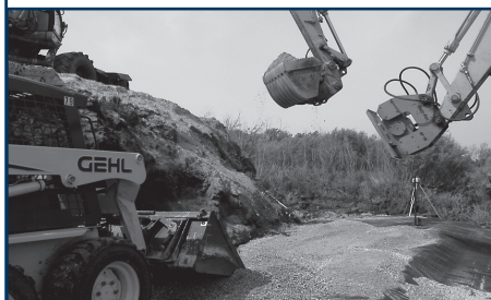
Leveling and compacting
