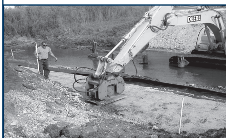
Compacting 8-in. lifts (Note: Pilings are vibrated in)
