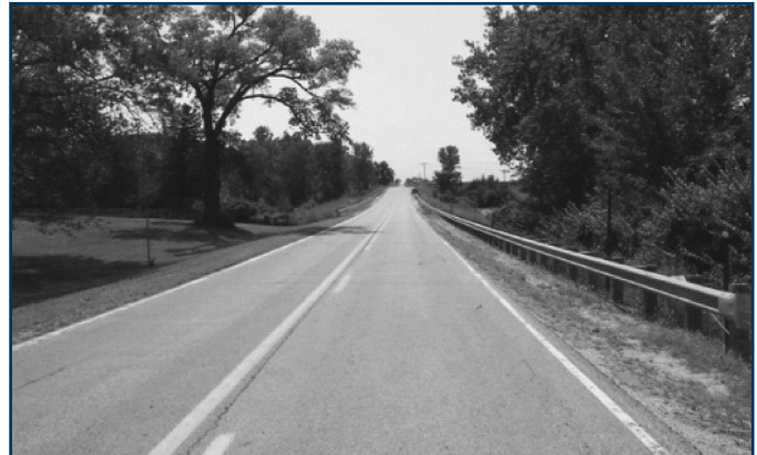
Guardrail along embankment at the edge of the county lake. (Photos courtesy of Bob Sperry)
