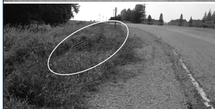
Cable guardrails at an embankment area (top) and at a curve location (bottom). (Photos courtesy of Tom McDonald)
