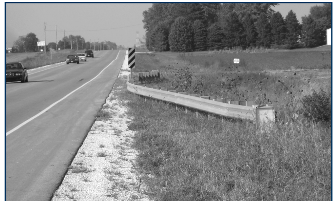
A guardrail around a culvert, protecting from the drop-off hazard. (Photos courtesy of Bob Sperry)
