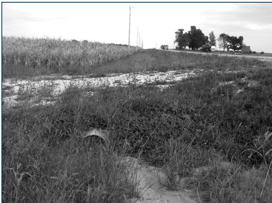
A flattened entrance slope with a culvert
