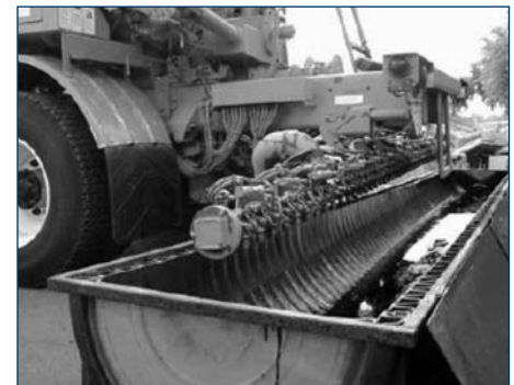
Figure 1. Distributor truck spray bars being emptied
