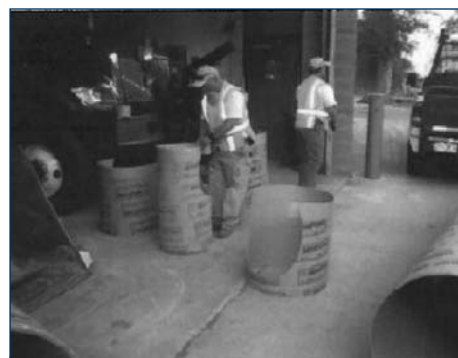
Figure 4. In-house construction of culvert
