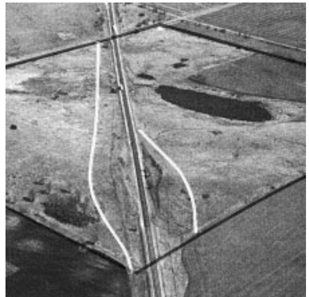
An aerial view of Engeldinger Marsh. The light colored lines show the approximate "footprint" of the proposed expansion of Highway 65.
