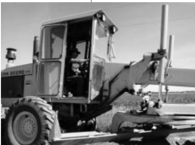
Keith Eppert, a Boone County motor grader, is hard at work.
