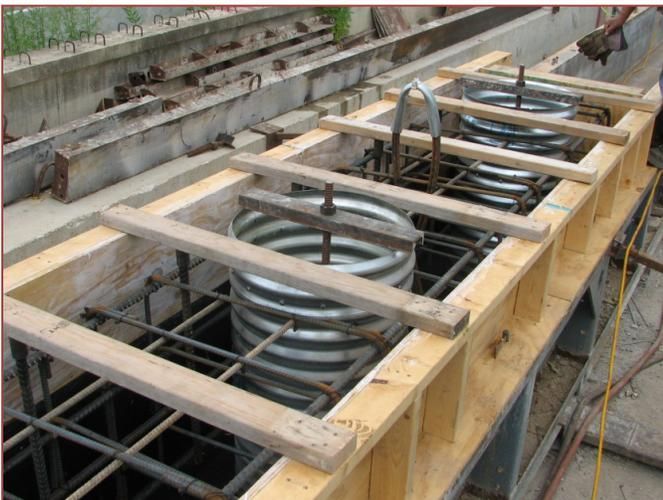
*Construction of abutment cap formwork showing one of the beam lift loops near one end of the form and two of the corrugated metal pipe (CMP) pile connection openings*
