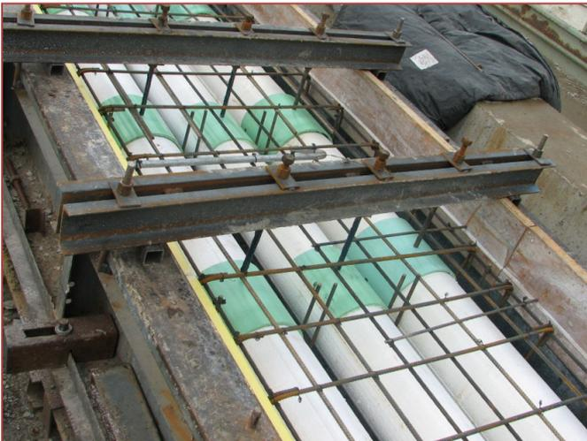
*Fabrication form setup for one of the seven precast/prestressed box girders/beams with Styrofoam cylinders used to create the voids*
