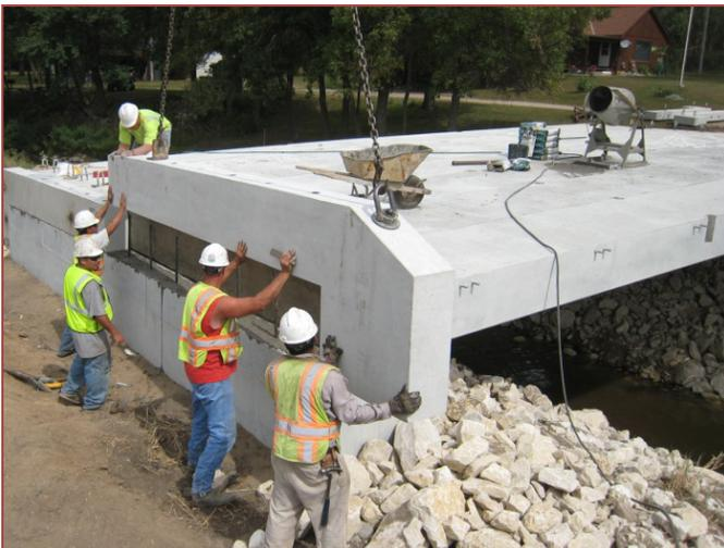
*Placement of second back wingwall onto anchor rods and epoxy grout bed on west end of bridge*
