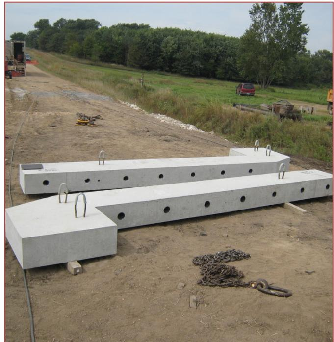
*Two of the four back wingwalls, each with three lifting loops and seven anchor rod openings*
