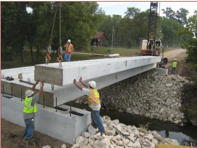
*Positioning exterior beam after extension of anchor rods along the edge of abutment caps and middle beam placement*
