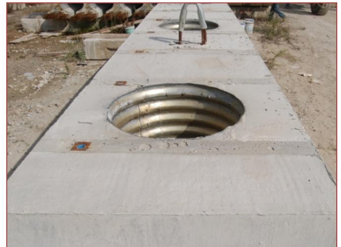
*One of the two precast abutment caps showing pile connection openings, guardrail post anchor rod extension openings along the edge, and one beam lift loop*
