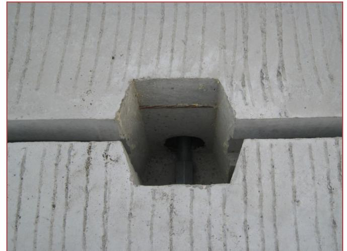
*Tie rod block outs in final precast beams for tightening the interior tie rods once bridge components are in place on site*
