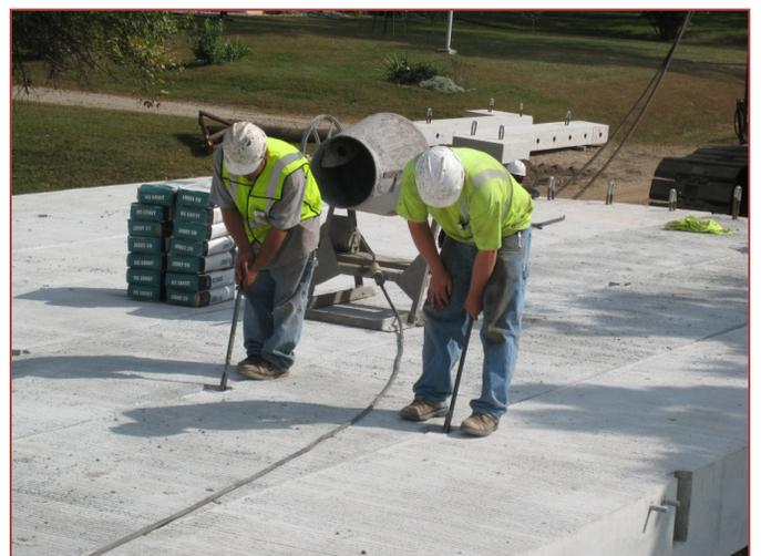
*Tightening transverse tie rods before filling block outs with epoxy grout*
