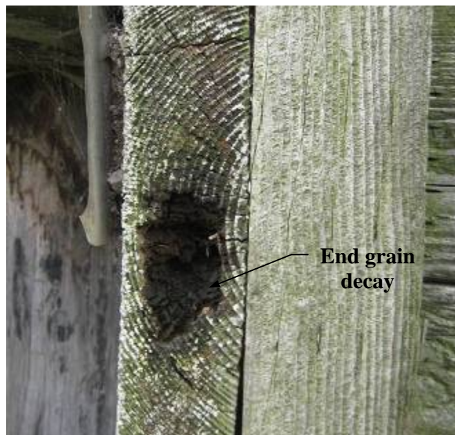
Figure 4-15. Poor end grain with decay was most common defect found in backwalls.
