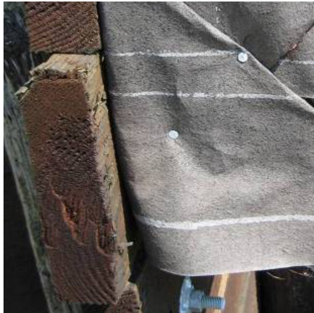
Figure 4-48. Good end grain treatment
