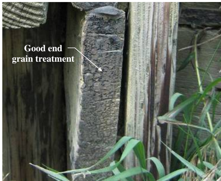
Figure 4-14. Good backwall with treated end grain
