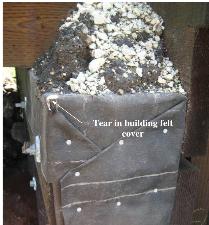
Figure 4-46. End of pile cap with building felt cover providing protection from moisture and weathering
