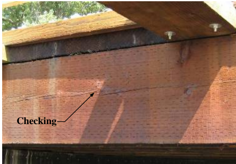
Figure 4-51. Exterior stinger with checking due to in-place seasoning
