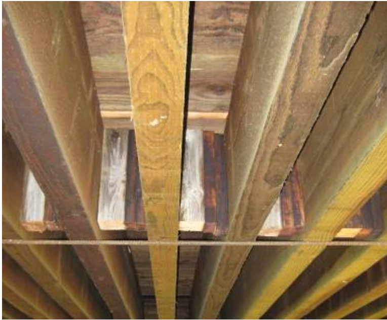
Figure 4-49. Good copper naphthenate-treated stringers
