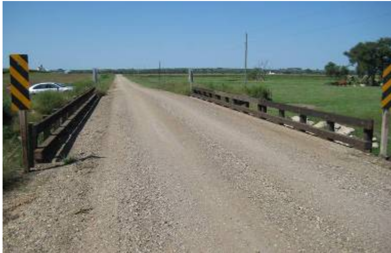
Figure 4-64. Good wearing surface protects the timber decking
