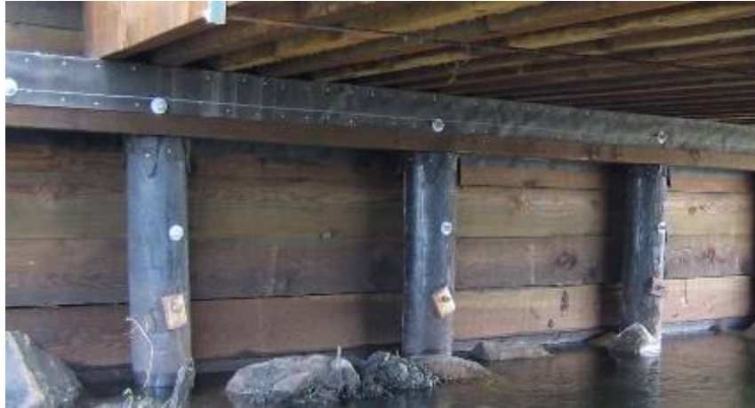
Figure 4-47. Good copper naphthenate backwall
