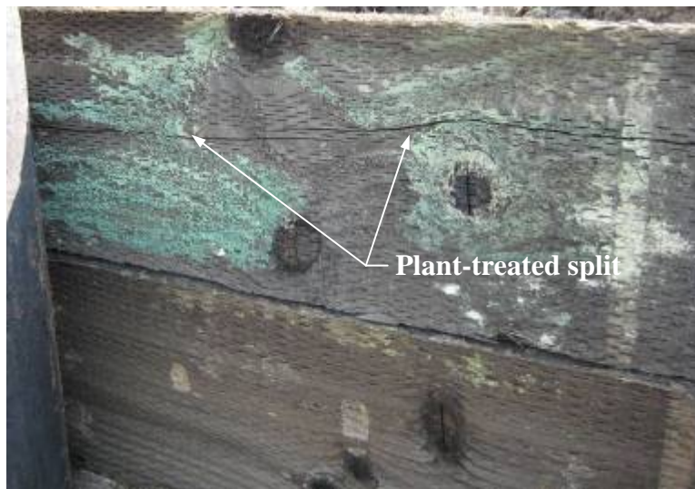
Figure 4-58. New ACZA treated back wall planks properly seasoned prior to treatment
