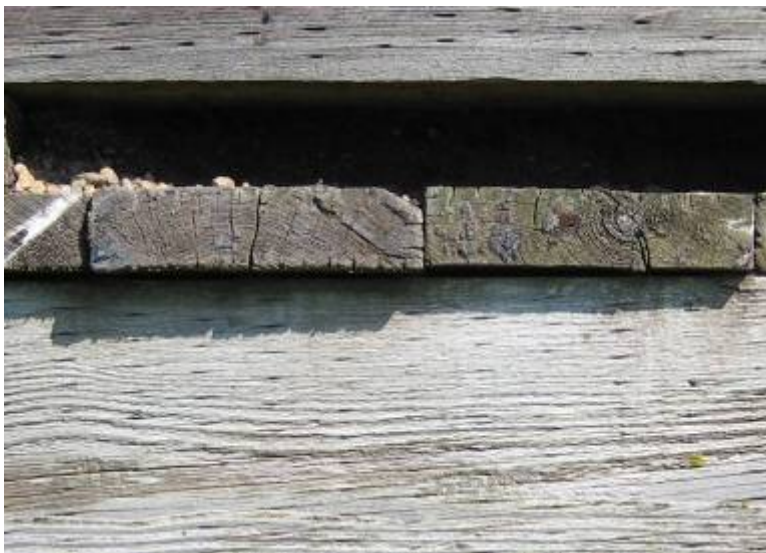
Figure 4-42. Physical defects at endgrain, ca. 1980
