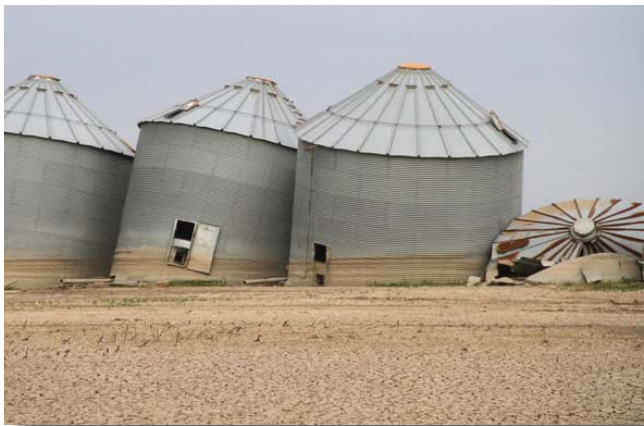
Damaged silos southwest of Hamburg in Fremont County. Photo from IUB website.
