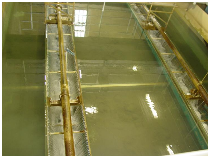
Observation of filter backwash cycle during filter media inspection
