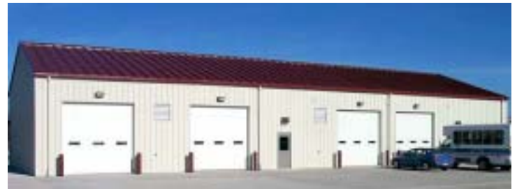
A 5,600 square foot transit storage facility in Jefferson helps to extend the life of aging vehicles. The facility can house six transit vehicles and allows for light maintenance. (South view of facility)
