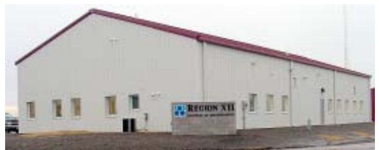
Greene County supported public transit by assisting with the land purchase and performing all site work for the project through the Secondary Roads Department. (Northeast view from intersection of Wall and Pinet streets in Jefferson)
