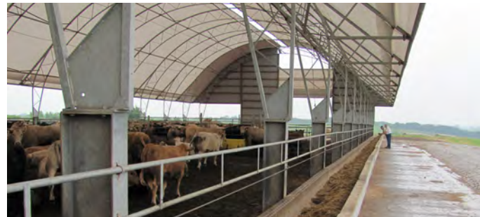
In Appanoose county, this feedlot was converted from an open lot to a roofed facility to eliminate manure runoff, with financing through the SRF LWQP.
