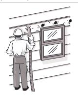
Although you may be able to rent the equipment for blowing insulation into your home's exterior walls, the job is very involved and is best handled by an experienced insulation contractor.
