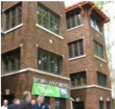
The newly-renovated Brown Apartments in Cedar Rapids
