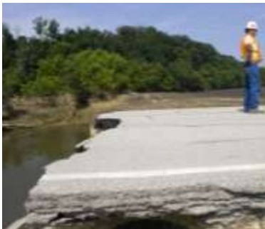
An Army Corps of Engineers employee stands on an Oakville road torn apart by flooding.
