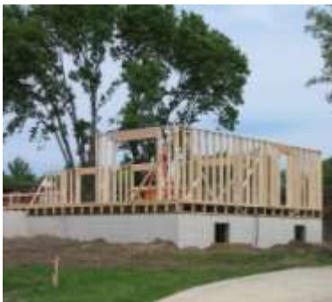
A home being constructed in Parkersburg
