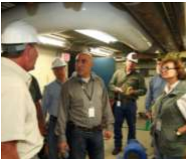
University of Iowa and FEMA officials review flooded ventilation, water and electrical systems.
