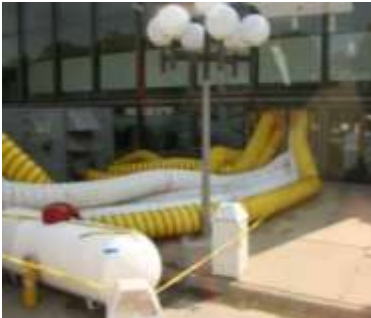
A flooded building at the University of Iowa dries after the flood water recedes in Iowa City.
