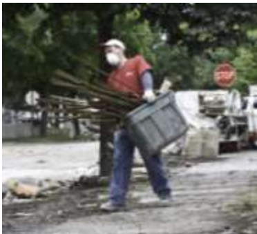
A volunteer clears debris from flooded homes in Cedar Rapids.
