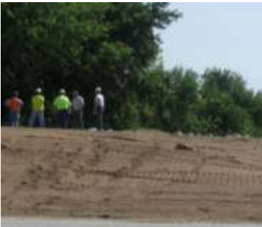
A levee being rebuilt near Oakville
