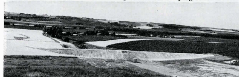
A gully control structure installed in the Nepper Watershed in the Little Sioux area to control a large gully which had progressed up through the farm land. Since this picture, the complete area has been treated and gully eliminated, as well as the farm land control being maximum conservation practices.
