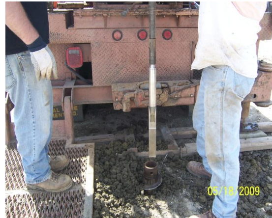
(b) Installing pressure cells
