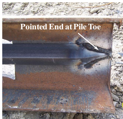
Figure 4.5. Angle bars were chamfered to form a pointed end at pile toe
