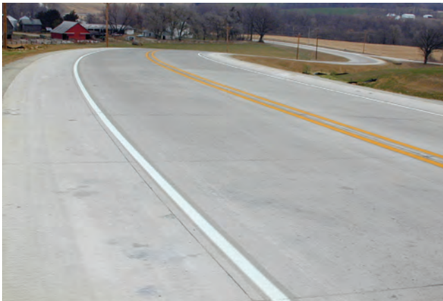
Figure 2-1. Unbonded overlay
