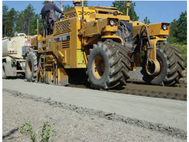
Figure 7-5. Mixing the cement into the pulverized material
