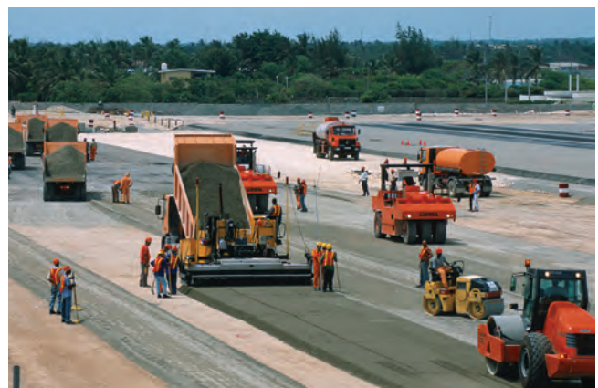
Figure 6-7. Placement of plant-mixed CTB on prepared subgrade
