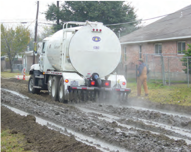
Figure 7-4. Applying cement slurry on grade prior to mixing (cement slurry is applied the same way for CTB applications)
