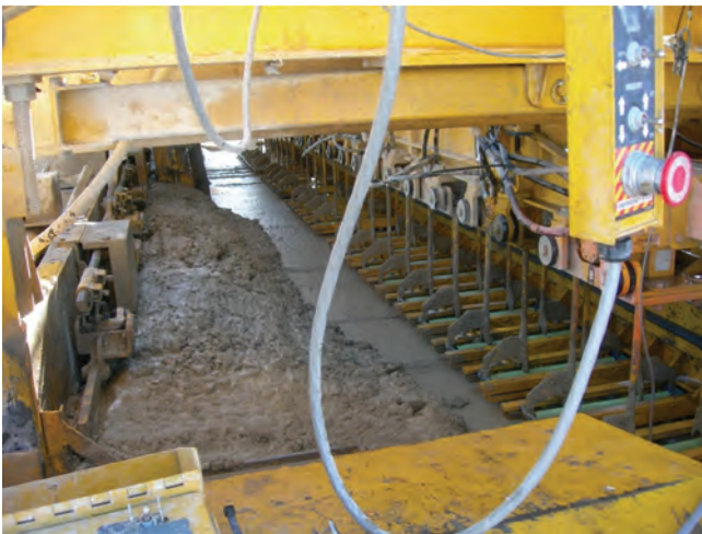
Figure 1-6. Dowel-bar inserter
