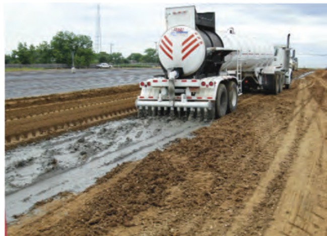
Figure 8-2. Cement slurry added to subgrade material (cement slurry is applied the same way for CTB and FDR applications)
