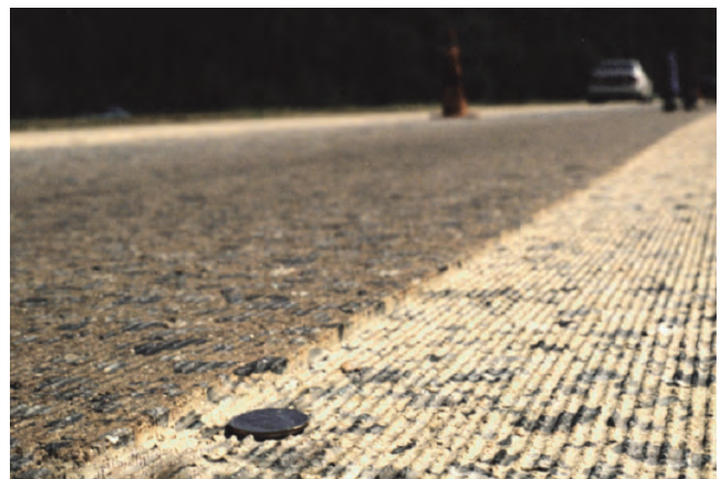
Figure 10-7 Diamond grinding concrete pavement for surface restoration
