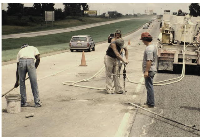
Figure 10-4. Drilling operation as part of slab stabilization
