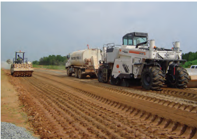
Figure 6-6. Constructing CTB using mixed-in-place method
