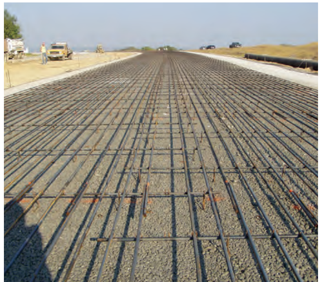
Figure 1-8. CRCP reinforcement placed before paving
