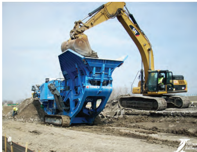
Figure 9-4. Existing concrete recycled in-place and reused for base material on the Tri-State Tollway in Illinois
