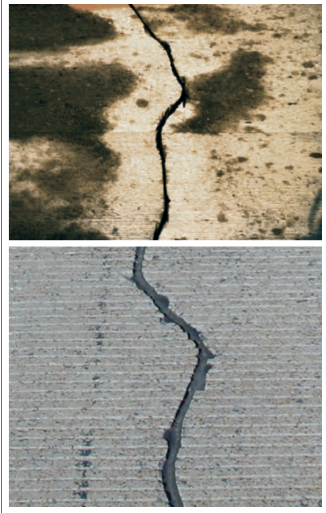
Figure 10-5. Application of joint sealant
