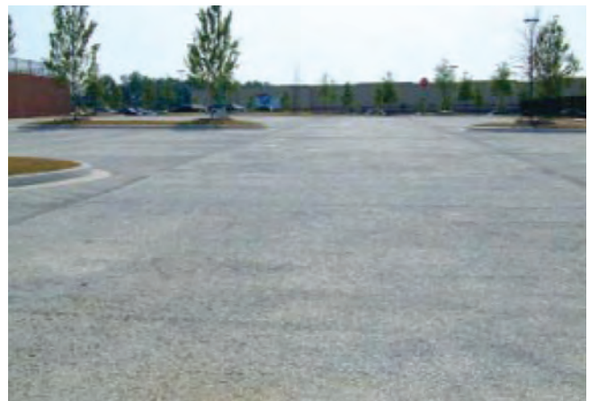
Figure 3-5. Pervious concrete pavement parking lot
