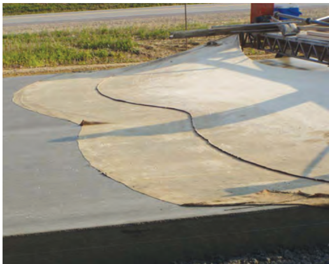
Figure 1-9. Burlap drag on fresh concrete
