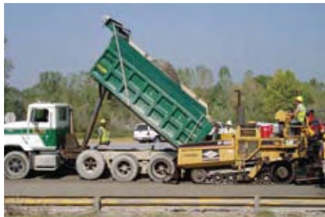
Figure 5-9. RCC delivered to jobsite
