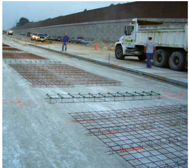
Figure 1-7. JRCP reinforcement in place before paving
