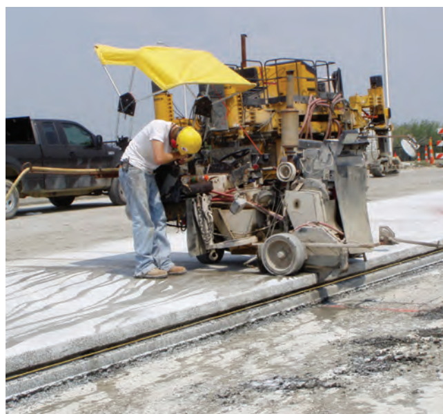
Figure 1-4. Sawcutting JPCP
