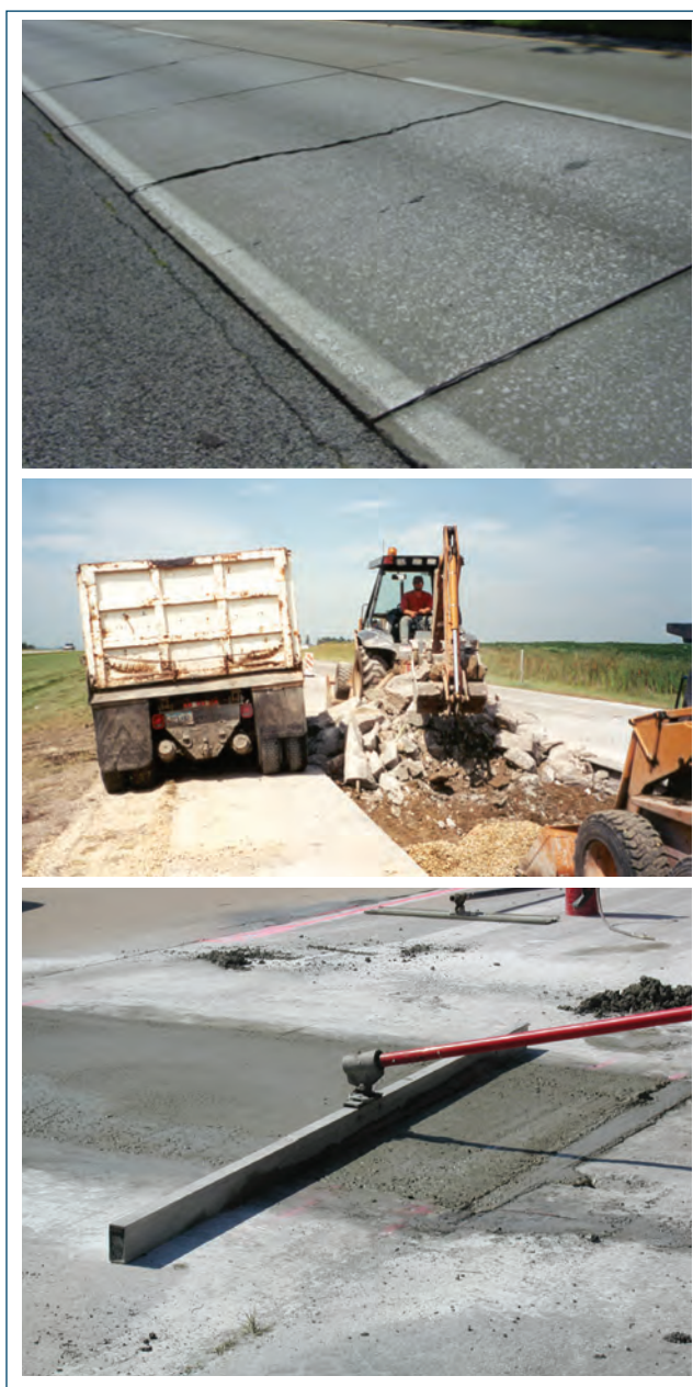
Figure 10-1. Full-depth repair of a concrete pavement slab
