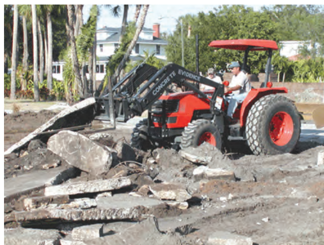
Figure 9-3. Broken concrete pavement is removed for recycling
