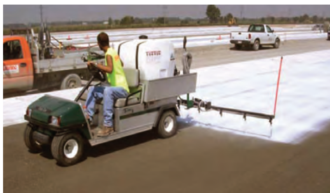
Figure 5-16. Curing RCC
