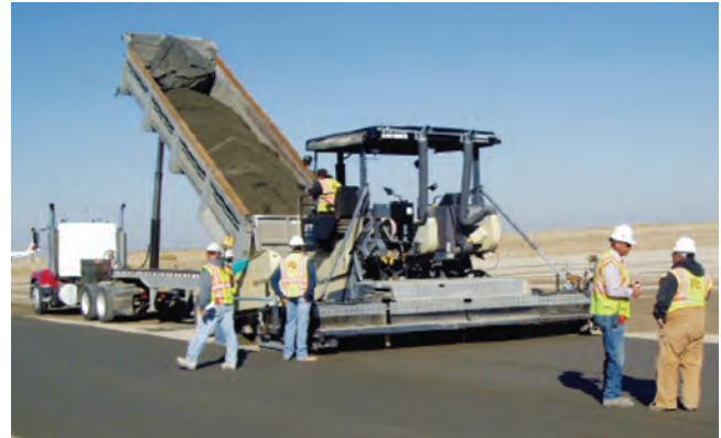
Figure 5-13. RCC placement
