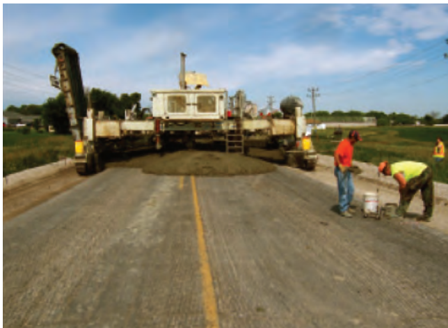
Figure 2-5. Bonded overlay construction
