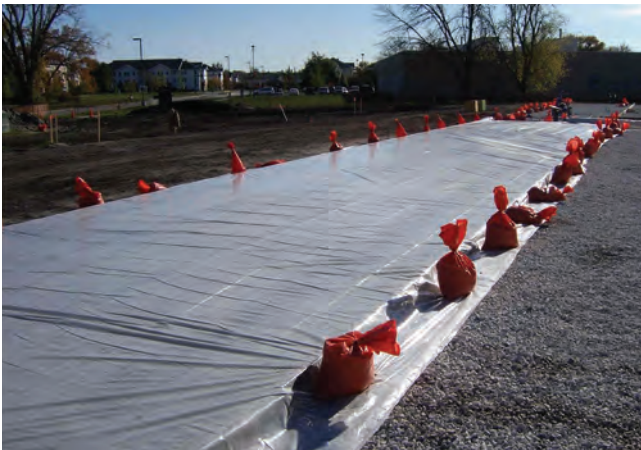
Figure 3-12. Curing pervious concrete with plastic sheeting
