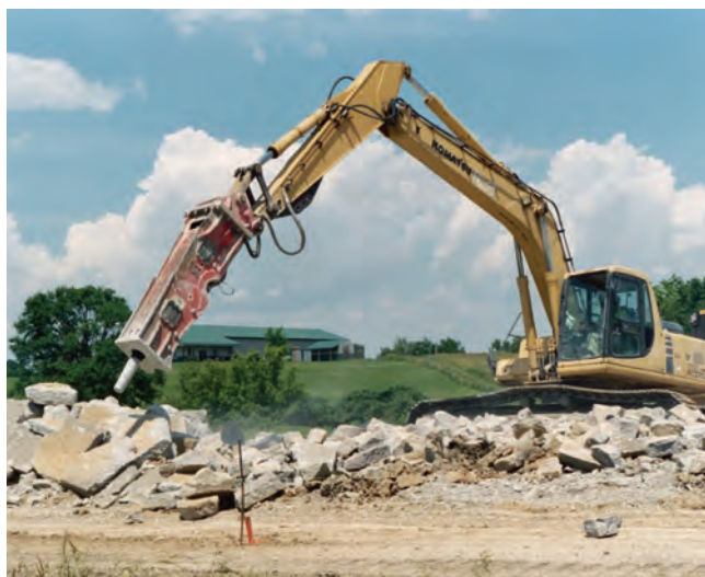
Figure 9-2. Example of equipment used to break existing concrete
