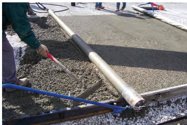
Figure 3-11. Compacting the placed pervious concrete
