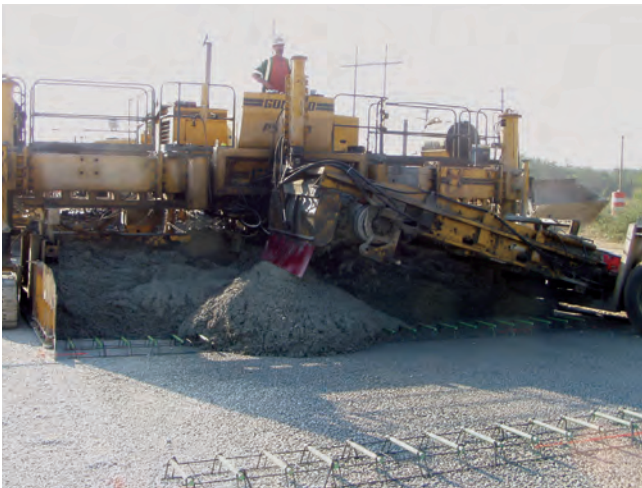
Figure 1-5. Concrete placed over dowel baskets
