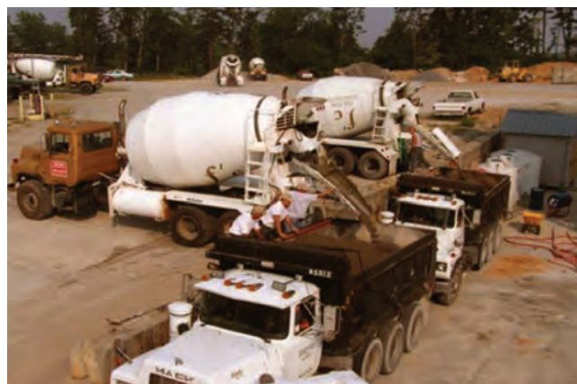
Figure 5-11 Ready-mix transit trucks dumping into haul trucks
