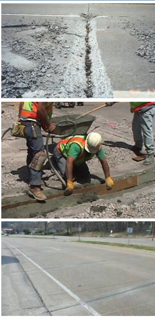
Figure 10-2. Partial-depth repair process at joint
