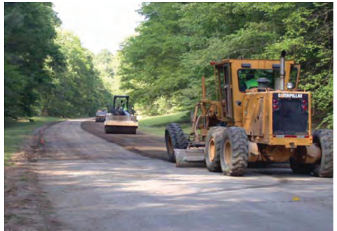
Figure 7-6. Equipment for compaction and finishing
