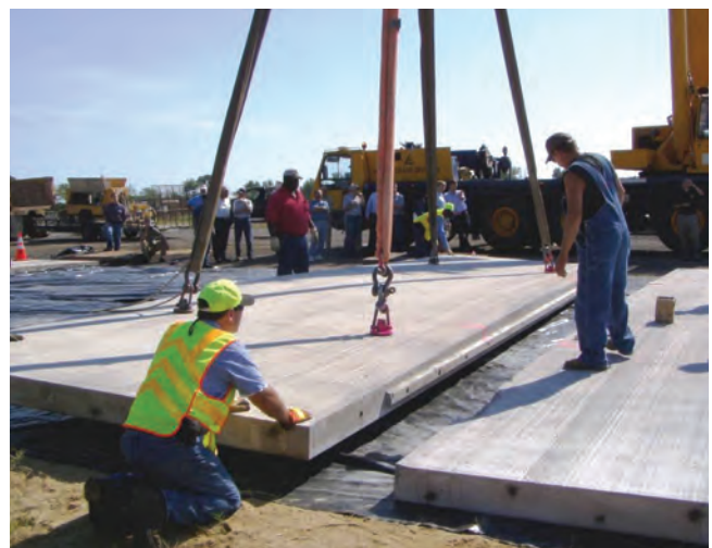
Figure 4-7. Placement of a prestressed precast panel
