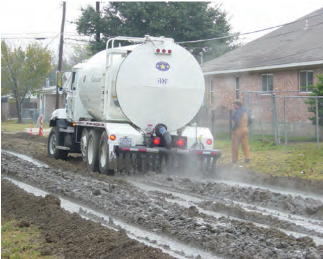
Figure 6-5. Applying cement slurry on grade prior to mixing (cement slurry is applied the same way for FDR and CMS applications)
