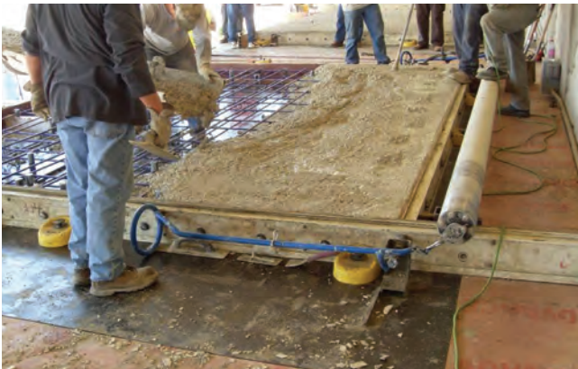
Figure 4-4. Concrete poured into form for precast panel
