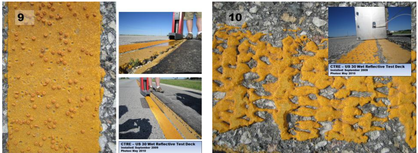
Figure 10. Ennis test sections 9 and 10 after one winter
