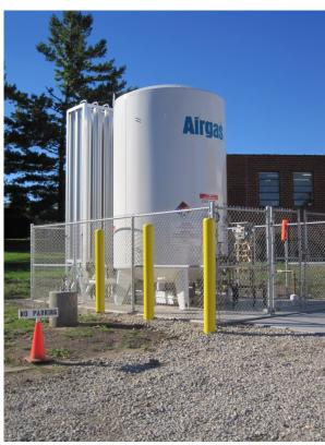
Oxygen tank no longer met code as it was too close to the building. Relocated tank to new, safer location across campus.
