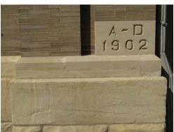
Tuck point all areas where mortar had decomposed and patch stone to ensure sound, weathertight building envelope.
