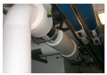
Water and sewer line replacement. Water and sewer lines were replaced in 2006. Most of the lines were close to 100 years old. Constant repairs to tiling needed to be completed to keep the lines open and operational. There was always concerns of water loss due to leaks and contamination of ground sewage lines.
