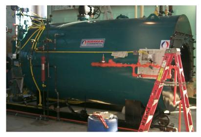
**Boiler replacement.** In FY2008 we used our routine maintenance funds to purchase and install a new summer boiler. The unit it replaced was decades old.
