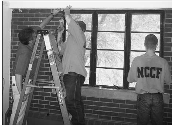
Production Coordinator Bob Mesecher supervises offenders installing window blinds at ISU.
