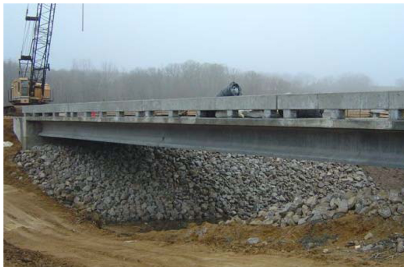
Elevation of Wapello County UHPC bridge during construction in 2005
