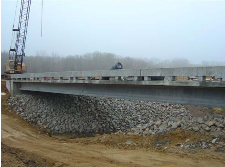
Figure 3.5. Elevation of Wapello County UHPC bridge.
