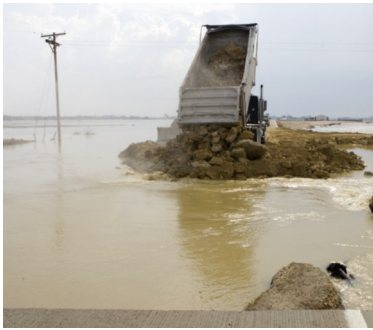
A truck dumps a load of rock into a levee breach in Oakville.
