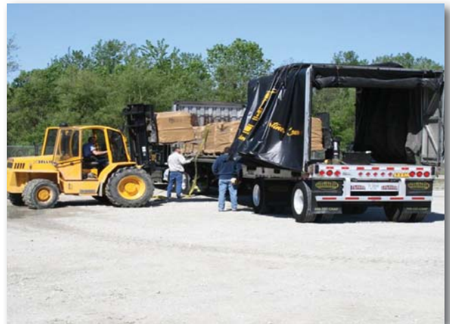
HSEMD and National Guard Staff load Hesco barriers bound for Louisiana. Photo by Joyce Flinn.
