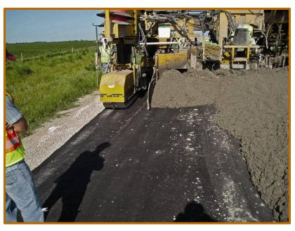
On County Road V-18 in Poweshiek County, a six-inch concrete overlay is constructed without the use of strings to control the paver. A fabric bond breaker between the new overlay and underlying pavement was used instead of the usual asphalt layer.
