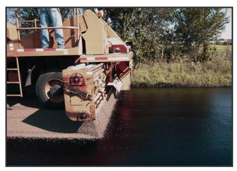
A chip spreader applies cover aggregate during a seal coat or "chip seal" operation on 74<sup>th</sup> Street in Cedar Rapids, Iowa, during a road maintenance effort *Photo: Dr. Charles Jahren, Iowa State University/CCEE*
