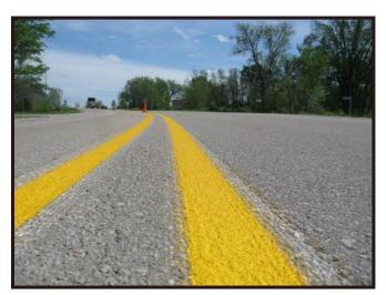
A pavement marking test deck in Dallas County, evaluating experimental centerline markings placed within a groove.
