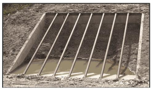
Safety treatment for cross-section drainage culverts *Photo: Midwest Roadside Safety Facility (MwRSF) University of Nebraska-Lincoln*
