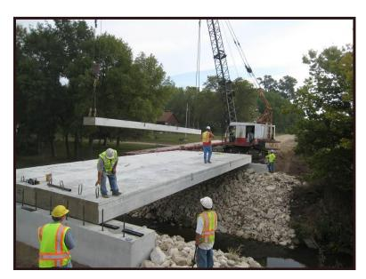
Beam placement during accelerated construction of Buena Vista IBRD bridge *Photo: Dr. F. Wayne Klaiber, Iowa State University/CCEE*
