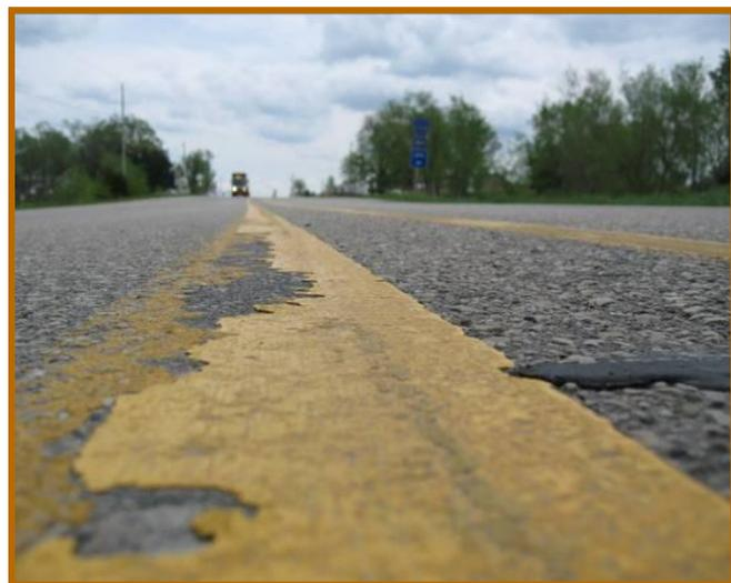
One goal of this project was to find new products and methods for improving both durability and retro-reflectivity of centerline markings.
