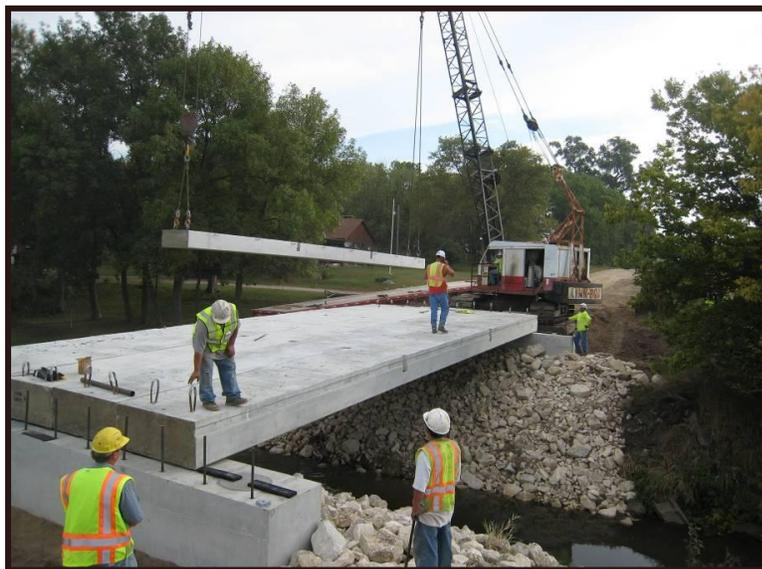
Beam placement during accelerated construction of Buena Vista IBRD bridge
