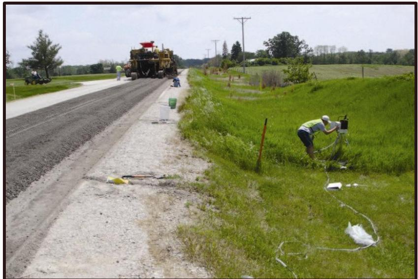
Installation of weather station
