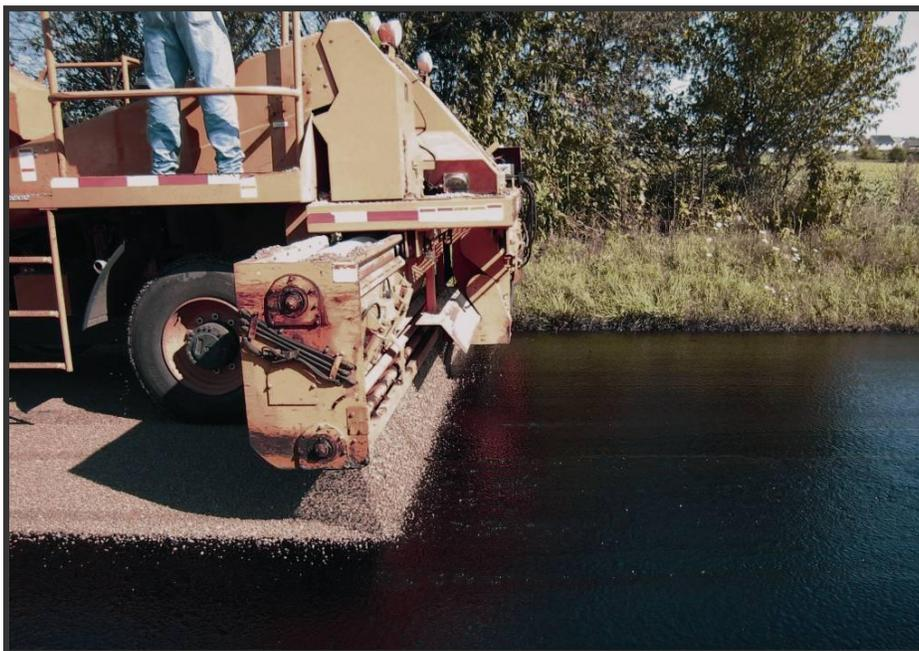
A chip spreader applies cover aggregate during a seal coat or "chip seal" operation on 74<sup>th</sup> Street in Cedar Rapids, Iowa, during a road maintenance effort
