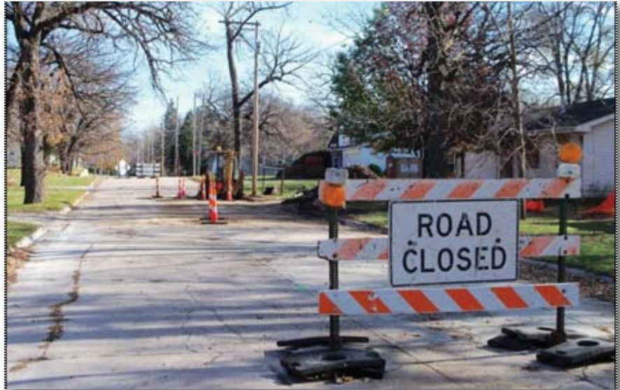
Severely damaged houses in Mason City slated for demolition. FEMA photo.
