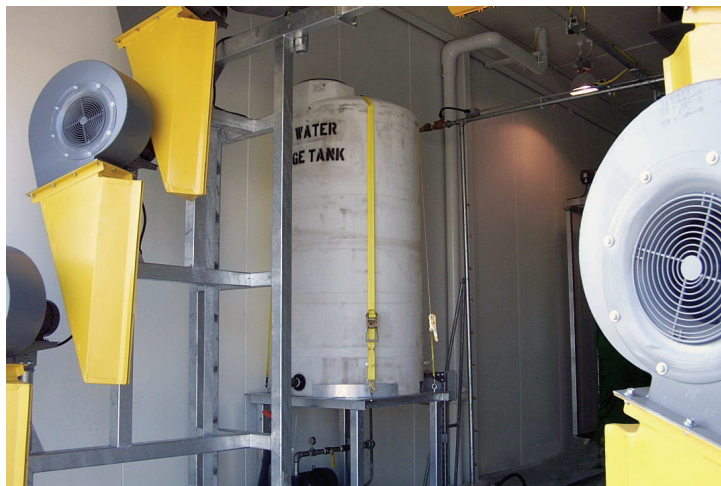
After each MTA bus is washed, 80% of the water is stripped off the bus by the bus dryer system.
