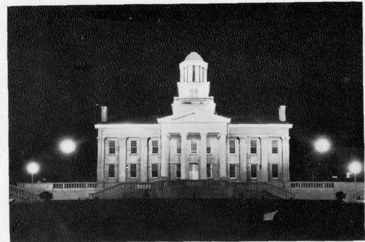
FLOODLIGHTS AT NIGHT ILLUMINATE IOWA'S MOST FAMOUS BUILDING
