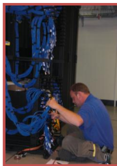
Jason Mease, ICN employee, making fiber/copper connections to the new Foundry Big Iron Ethernet Switch.
