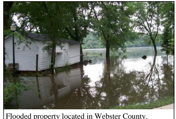
Flooded property located in Webster County.
