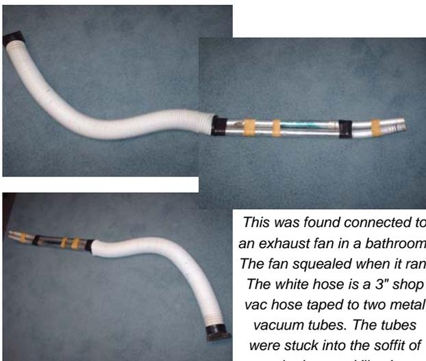
*This was found connected to an exhaust fan in a bathroom. The fan squealed when it ran. The white hose is a 3" shop vac hose taped to two metal vacuum tubes. The tubes were stuck into the soffit of the house... Yikes!*
