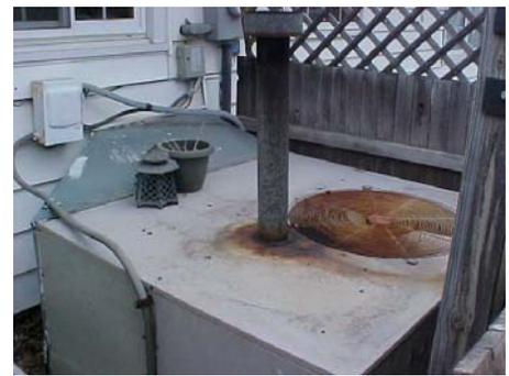
This is a picture of a furnace and air conditioning combination that is an outside unit. The day before, MEC had been to the home and didn't test for CO. They told the client the furnace was simply not running well. When Threshold arrived and tested the stack CO, they found it was over 1800 ppm.
