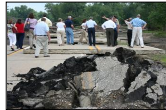
Members of the Rebuild Iowa Advisory Commission survey a roadway heavily damaged by floodwaters near Oakville.
