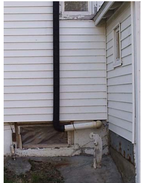
The hot water heater flue in the basement is metal going into PVC through the foundation and up through a corrugated plastic drain tile. It reconnects to metal at the top. Who knows what is coming out of the ground. The furnace is a 90% and does not draft through this pipe.
