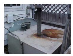
This is a picture of a furnace and air conditioning combination that is an outside unit. The day before, MEC had been to the home and didn't test for CO. They told the client the furnace was simply not running well. When Threshold arrived and tested the stack CO, they found it was over 1800 ppm.
