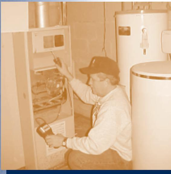
Professionally trained technicians in the program use a computerized energy audit to determine the most appropriate and cost-effective energy-saving measures that should be applied to the house. Typical measures include sealing air leaks, installing insulation in attics, walls, and crawlspaces, tuning and upgrading heating systems, and installing low-cost energy conservation measures.
