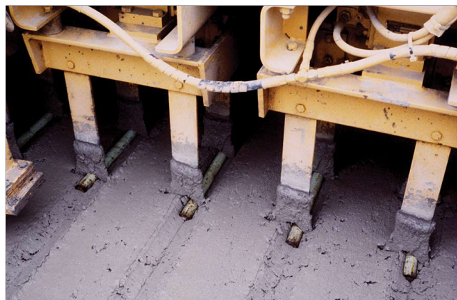
Figure 8-13. Dowel bar insertion equipment (ACPA)
