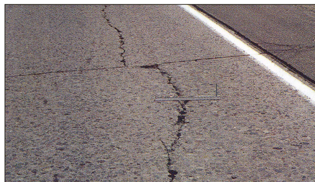
Figure 5-34. Random longitudinal crack
