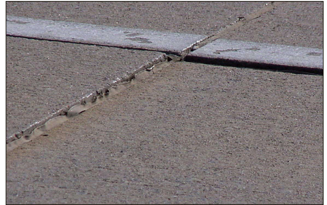
Figure 2-8. Faulting in jointed concrete pavement (ACPA)
