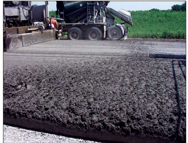
Figure 5-1. Segregated concrete (Hanson, Iowa DOT)
