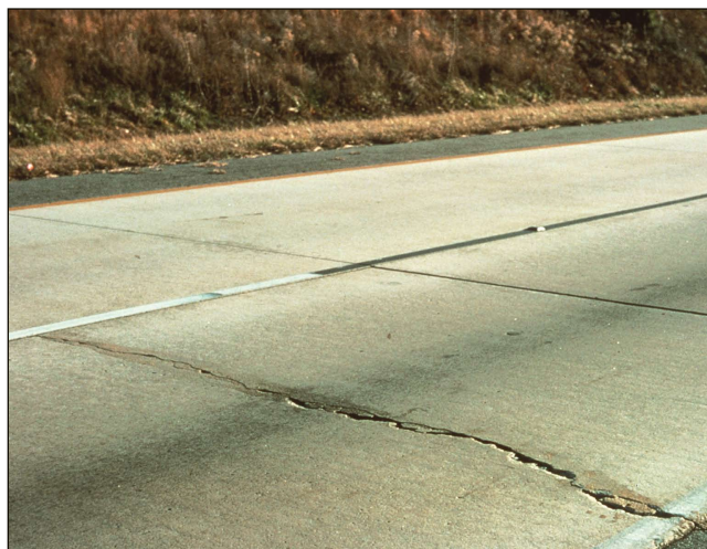
Figure 2-5. Transverse crack that represents structural distress (ACPA)
