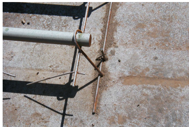
Figure 8-12. (a) Staking or (b) pinning dowel cages (ACPA)
