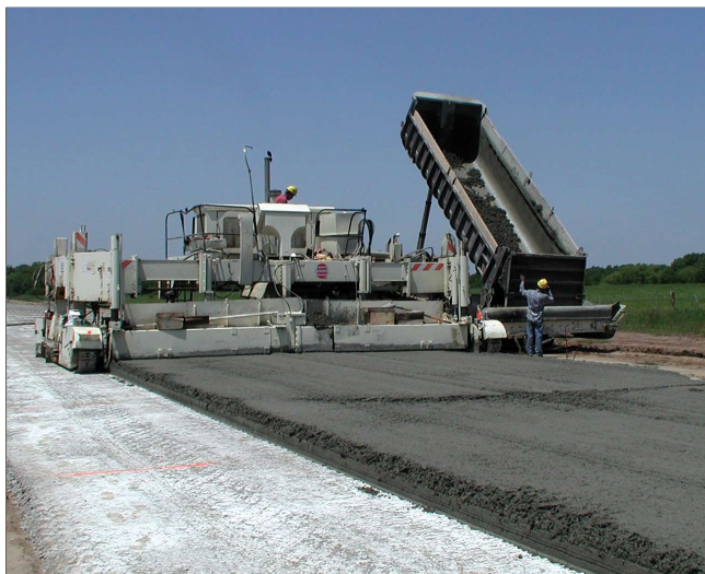
Figure 8-6. A belt placer/spreader ensures a consistent amount of concrete in front of the paver. (ACPA)
