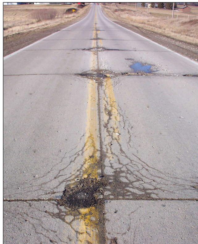
Figure 3-11. D-cracking (Jim Grove, CPTech Center)
