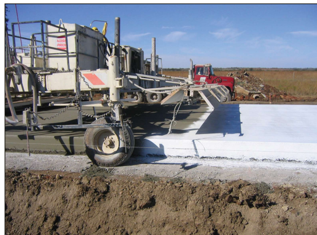
Figure 8-15. A curing machine coats both the top surface and sides of a slipform paving slab. (ACPA)
