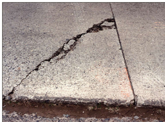
Figure 2-4. Corner cracking in jointed concrete pavement (ACPA)
