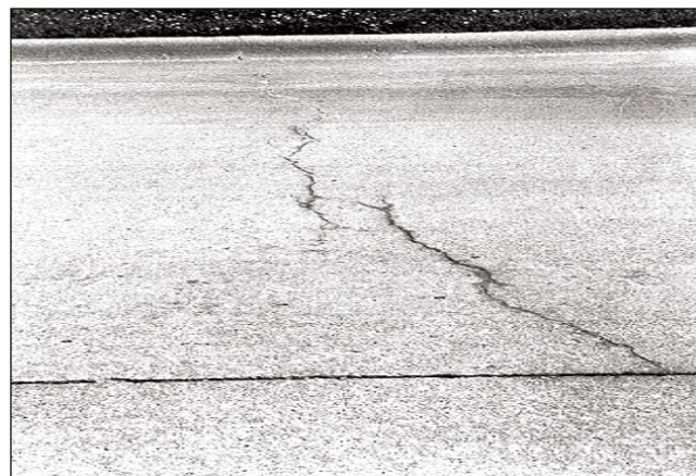
Figure 5-33. Random transverse crack
