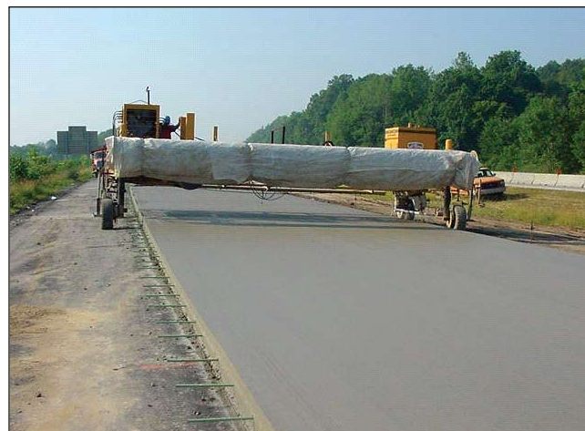
Figure 8-17. Plastic sheeting ready for placement to protect the fresh surface from rain (ACPA)
