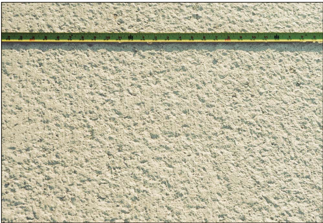
Figure 8-18. Typical scaling of concrete pavement due to rain on nondurable paste surface (ACPA 2003a)
