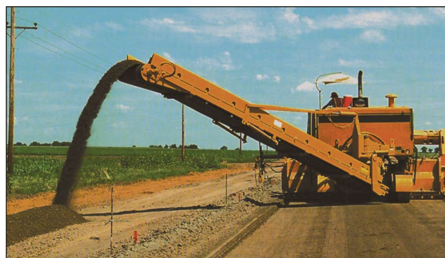
Figure 7-3. Autograder that references the string line and trims the subgrade material (ACPA)
