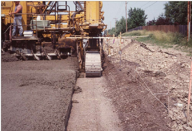
Figure 7-4. Trackline of slipform paving machine (ACPA)
