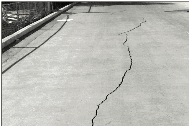
Figure 2-6. Longitudinal crack representing structural distress (ACPA)
