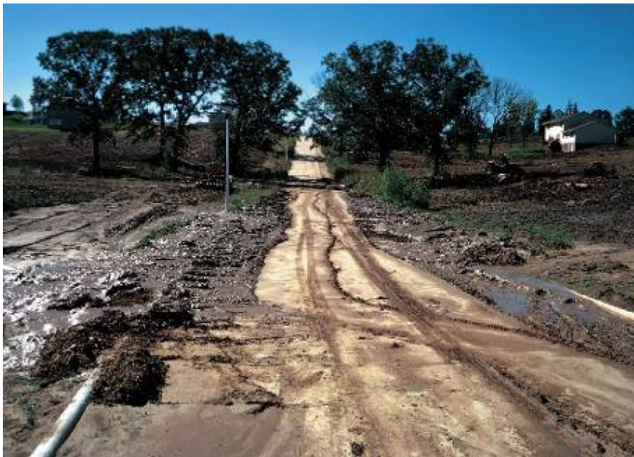
Figure 1: Sediment in street due to inadequate erosion and sediment control during construction
