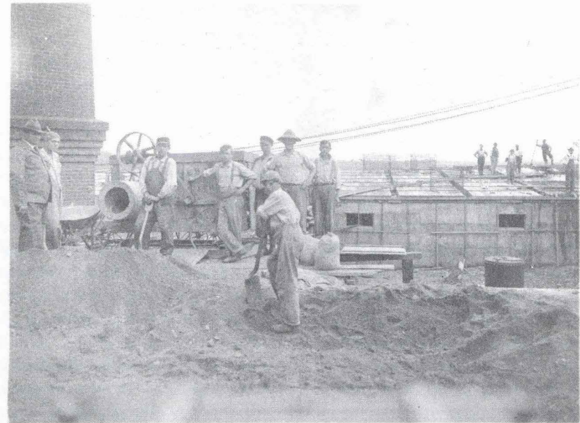
Constructing a Coalbin
