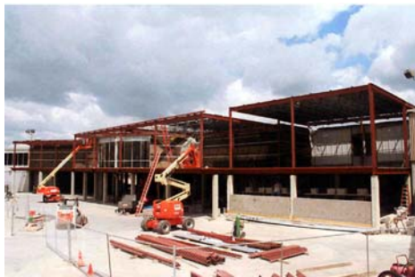
The concession expansion taking place on the Concourse level of the Terminal
