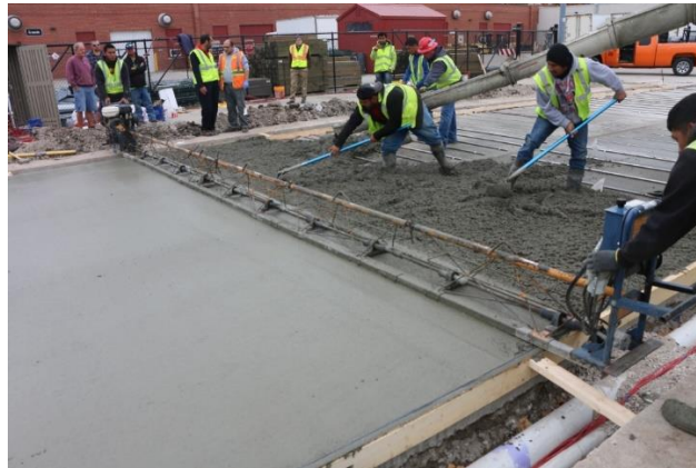
Figure A-2. ECON construction procedure
