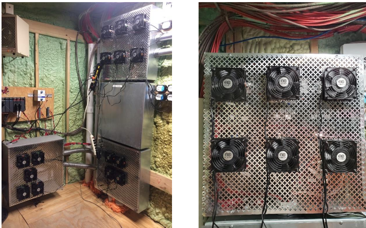
Figure 33. Cooling fans installed on the relays
