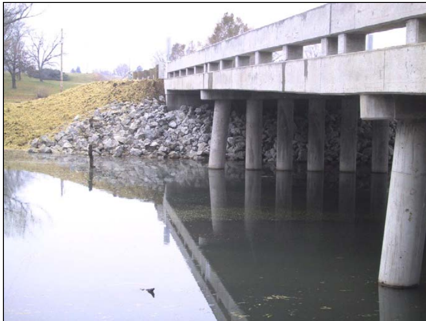
Figure B-8. Riprap abutment protection for a new county bridge; Pike Run Creek in Muscatine County, Iowa
