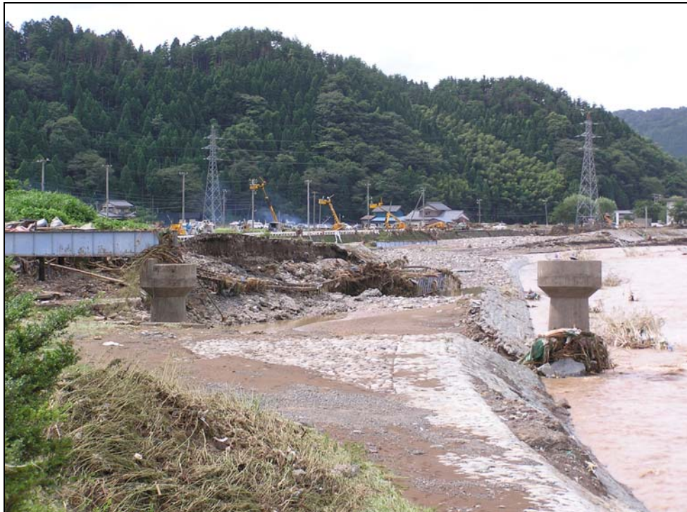
Figure A-14. Pier scour in floodplain, Asuwa River, Japan (courtesy of Prof. T. Hosoda, Kyoto University)
