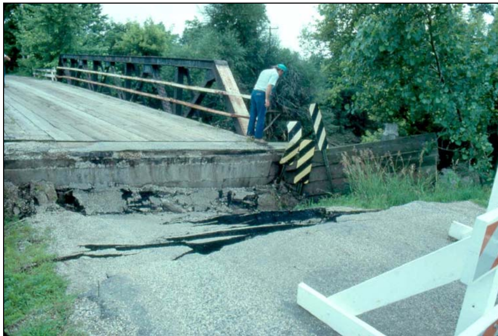
Figure 1-3. Collapse of a road embankment at a small bridge in western Iowa
