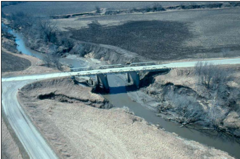
Figure 2-2. General degradation, associated with stream-bed head-cutting threatens the stability of piers and abutments of a bridge in western Iowa
