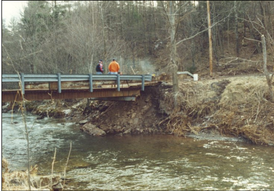
Figure 7-1. Basic monitoring of a small bridge entails observing conditions at the site, as well as upstream and downstream of the bridge site
