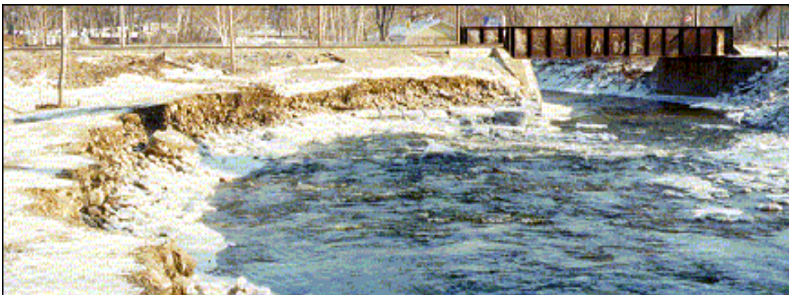
Figure A-3. Eroded left bank – unknown river
