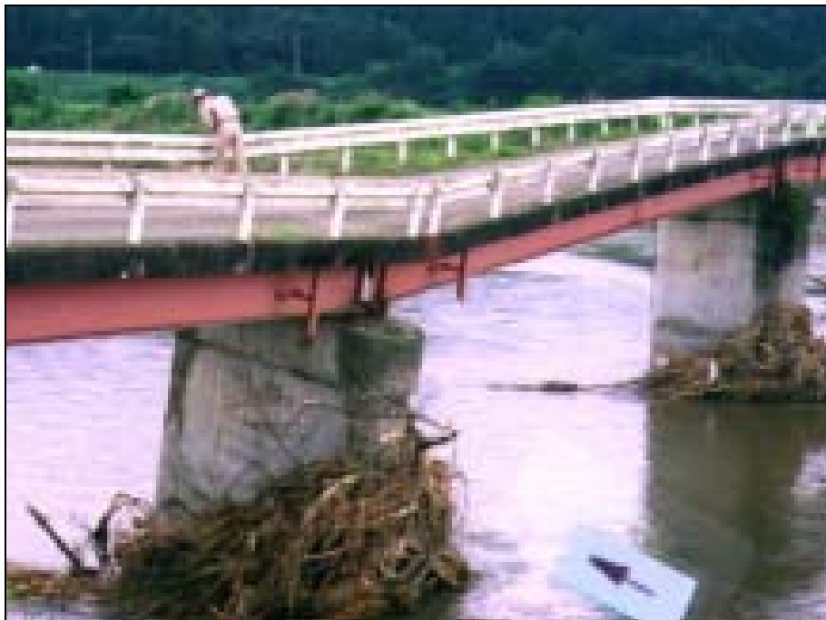
Figure A-18. Pier scour – Abukuma River, Japan (courtesy of Prof. T. Hosoda, Kyoto University)
