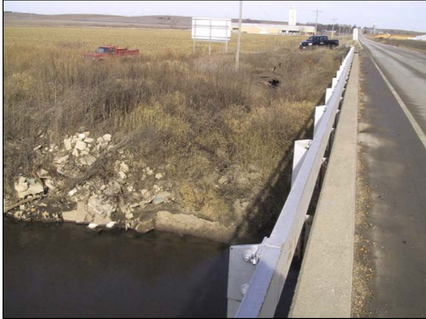
Figure B-17. Protection of lateral drainage using construction debris for Highway N16 bridge, East Nishnabotona River in Cass County, Iowa
