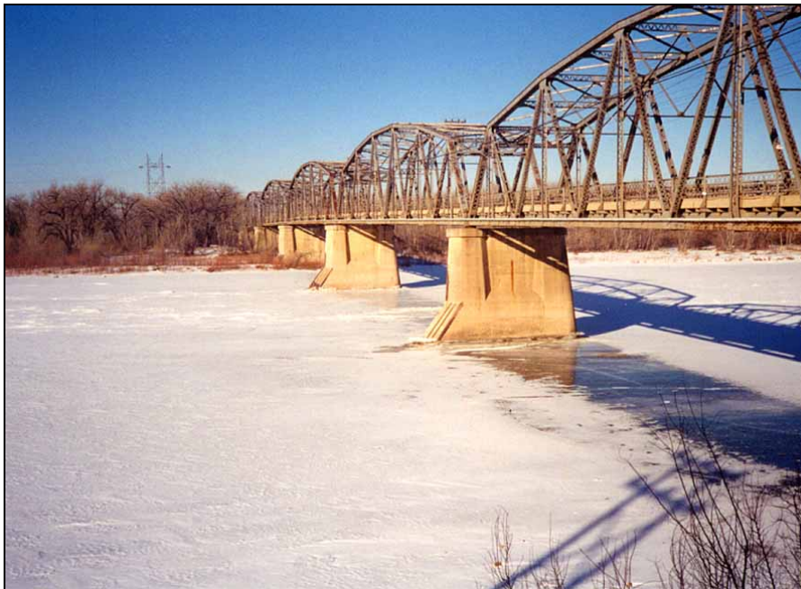
Figure B-12. Sloped nose of pier reduces ice loads on pier, and deflects ice from pier; Yellowstone River, Montana
