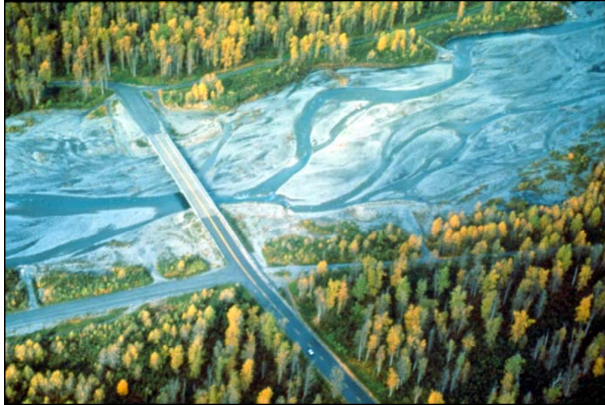
Figure B-18. Use of guidebanks fitted around abutments of a bridge over a braided channel; Lowe River, Alaska
