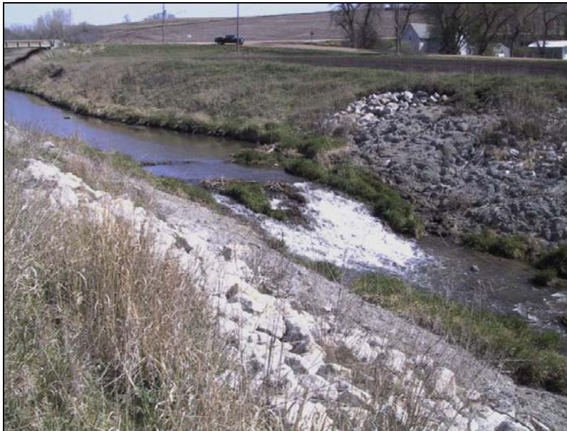
Figure B-39. A rock weir provided below County Road bridge on E16 to stop knickpoint migration, Porter Creek in Crawford County, Iowa -- notice that riprap is protected with grout so that rocks will not be dislodged during high flows
