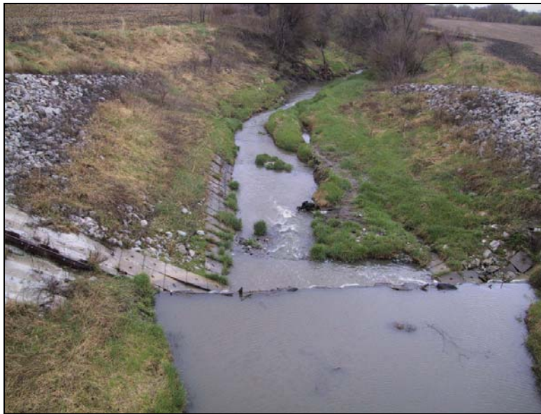
Figure B-36. A sheet-pile weir fortified with riprap downstream from County Road F52 bridge, Pigeon Creek in western Iowa
