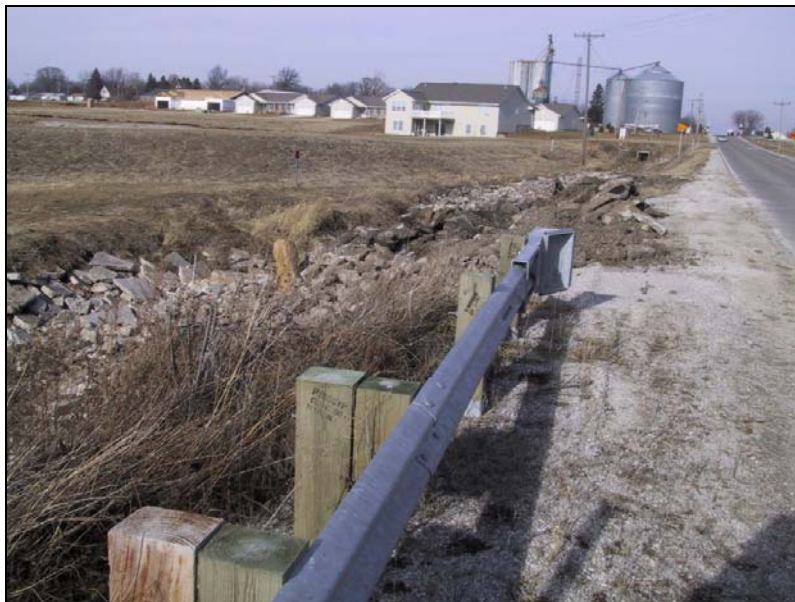
Figure B-16. A close-up view of head cutting protection of lateral drainage in Y26, Mud Creek in Muscatine County, Iowa
