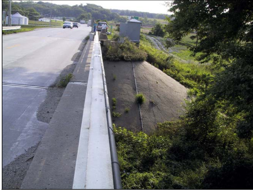
Figure B-7. Concrete-lined spill-through abutment protection for US Highway 137 bridge; Des Moines River in Wapello County, Iowa
