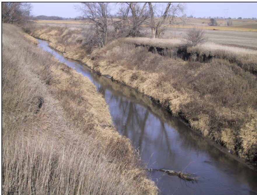
Figure A-5. Failed left and right banks upstream of bridge, Walnut Creek on G66, Iowa
