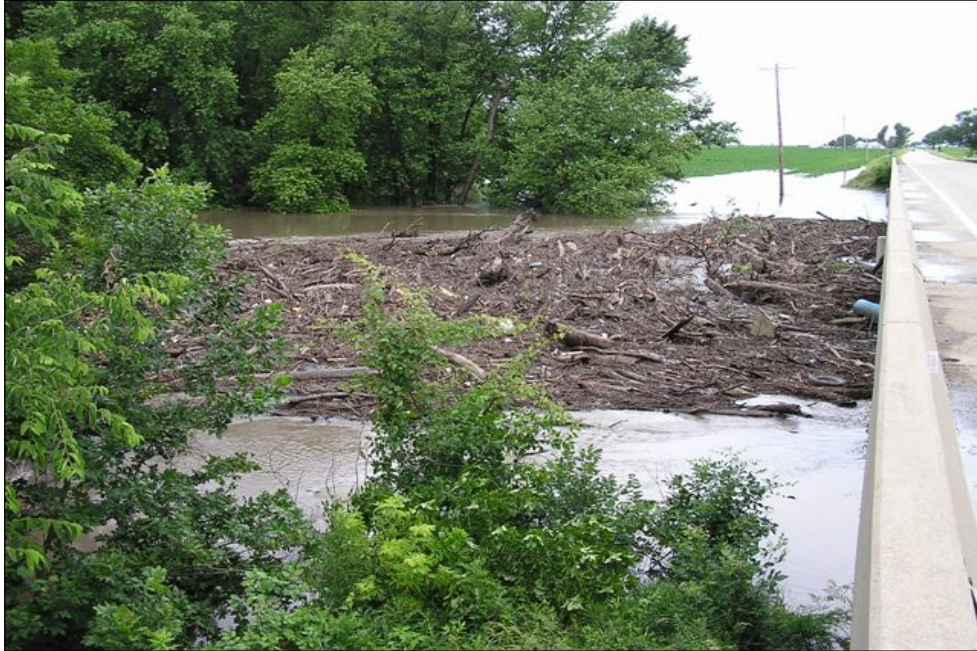
Figure A-36. Debris accumulation at piers, Iroquois River, Illinois
