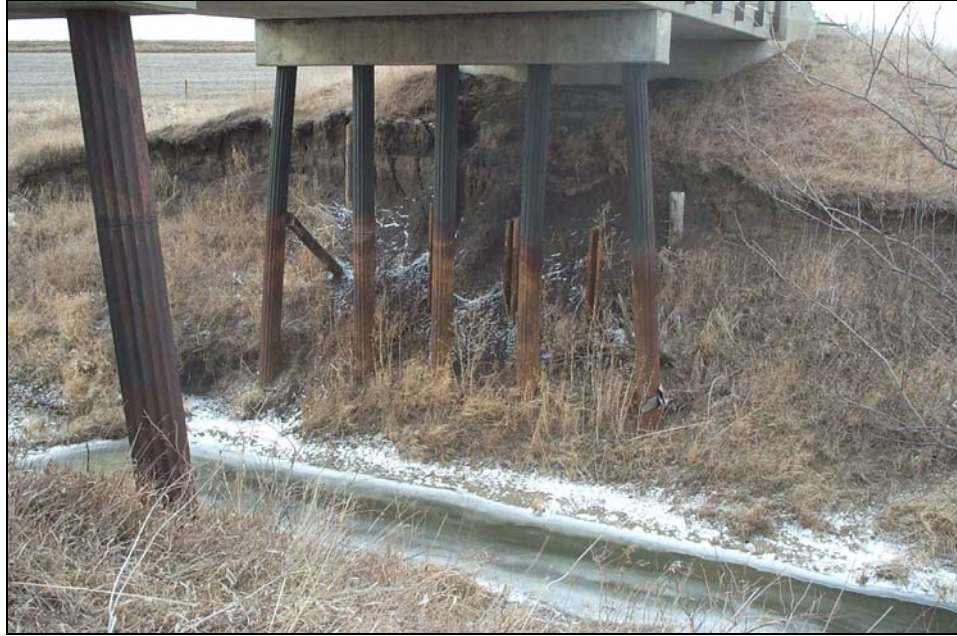
Figure A-13. Pier scour associated with channel degradation – unknown river in Iowa
