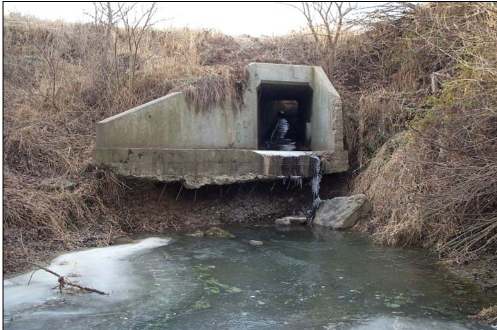
Figure A-47. Deep scour hole created downstream of culvert outlet – culvert in Iowa
