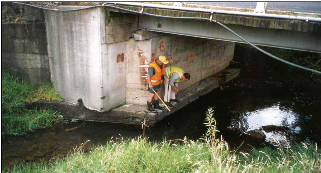
Figure 1-2. Bridge-inspection personnel checking for scour beneath the pile cap of a vertical-wall abutment
