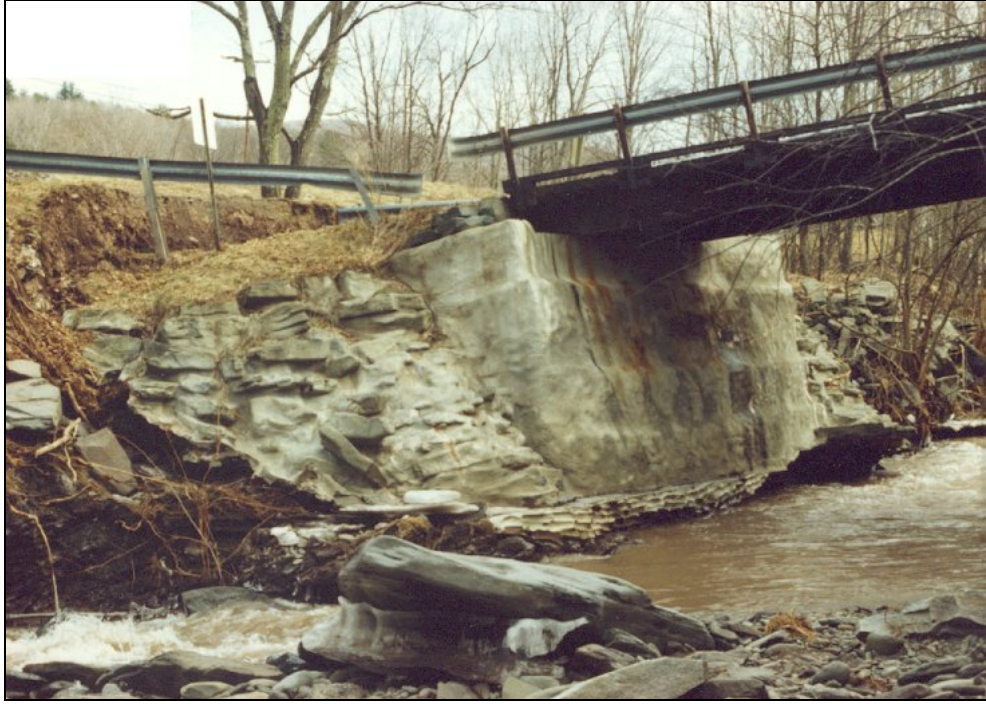
Figure A-25. Cuspate embankment failure of abutment on rough footing, Shoemaker Creek, New York
