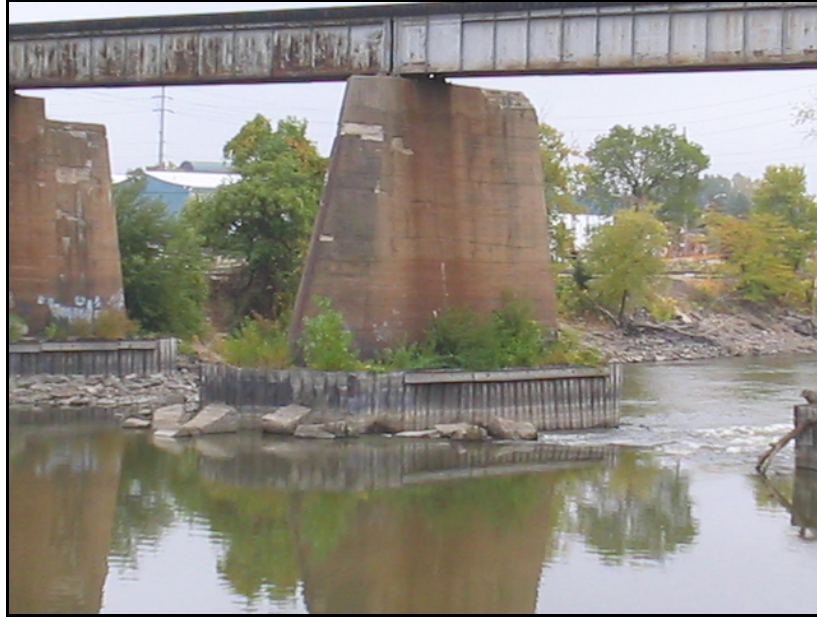
Figure B-3. Sheet piling placed around pile footing of a railway bridge pier in a channel that has lowered by general bed degradation, Iowa River in Iowa City, Iowa, below Coralville Reservoir. The leading edge of the sheet piling is protected with large blocks of stone and concrete.
