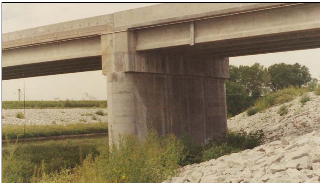
Figure B-33. The repair of the abutment scour shown in Figure 5-23 entailed adding a span and moving the abutment back up the channel bank; Boyer River, Iowa
