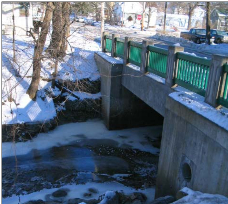
Figure A-45. Local scour at downstream side of vertical-wall abutment due to wake eddies associated with flow separation from abutment, Ralston Creek, Iowa City, Iowa
