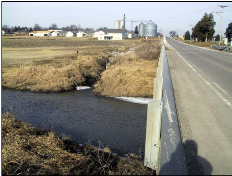
Figure B-15. Head-cutting protection of lateral drainage in Y26, Mud Creek in Muscatine County, Iowa
