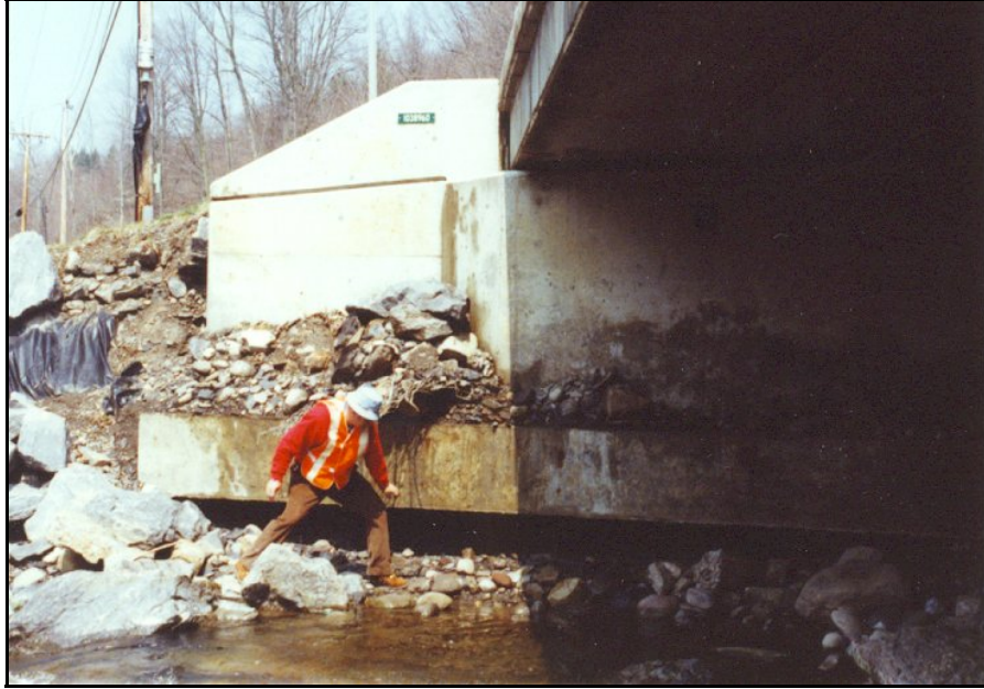
Figure 5-1. Inspecting pile exposure at an abutment after a flood-flow event, Fullmer Creek, New York
