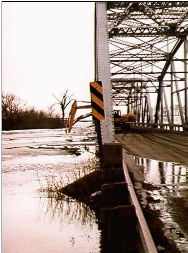
Figure B-14. Use of a backhoe for removing ice; Red River, North Dakota
