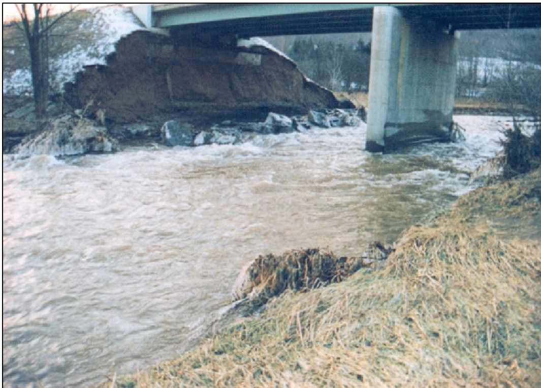
Figure A-28. Bank failure at abutment, Plate River, New York
