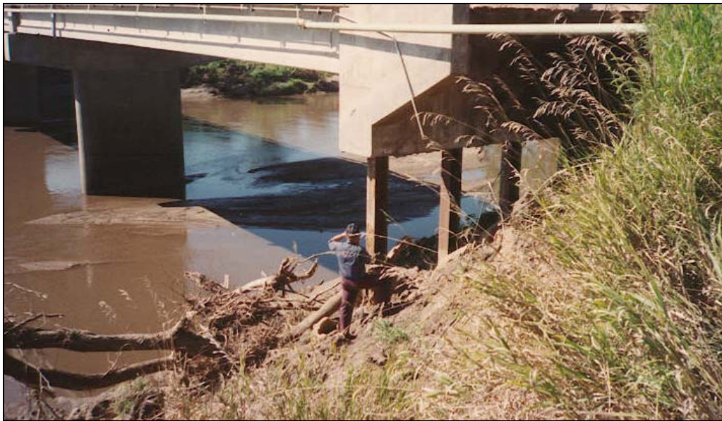
Figure A-23. Embankment erosion, exposing abutment piling, Boyer River, Iowa
