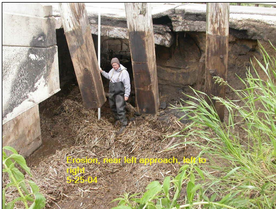
Figure 7-5. Measurement of erosion extent behind a wing-wall abutment, Turkey Creek, Iowa
