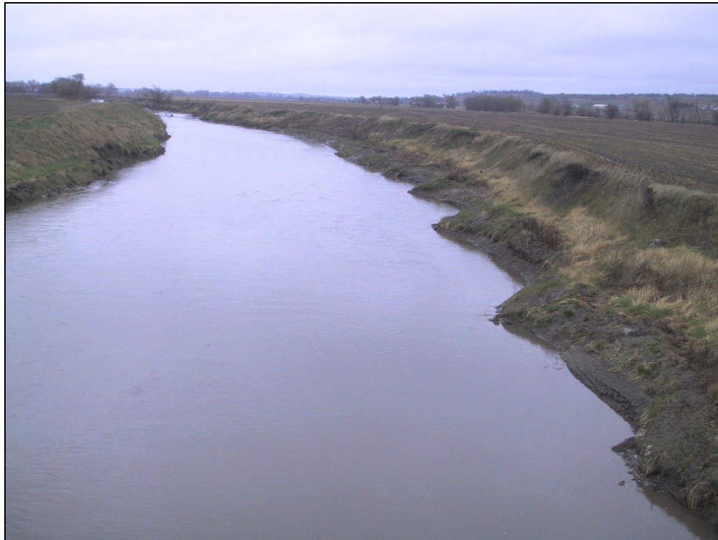
Figure B-24. Hard points installed along the concave bank upstream from Highway 37 bridge; Boyer River near Dunlap in Crawford County, Iowa
