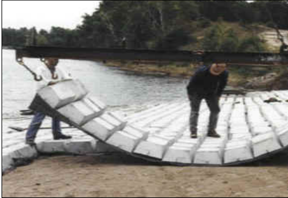
Figure B-30. Prototype installation of cable-tied blocks near an abutment –unknown river, New Zealand
