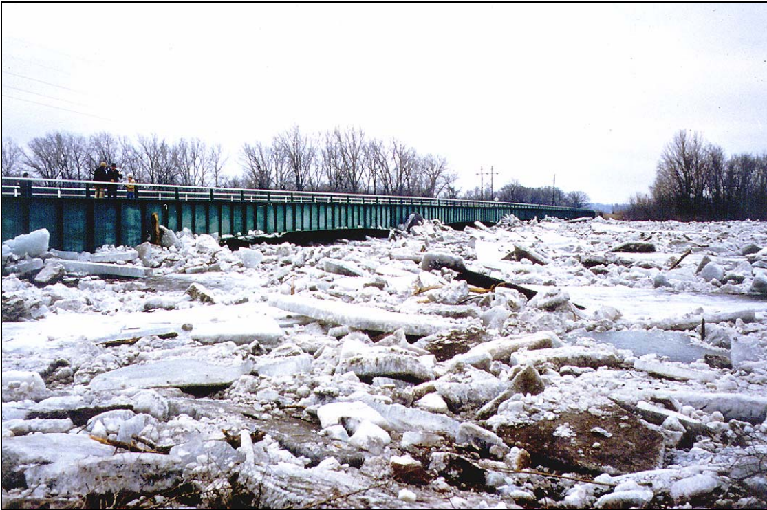
Figure A-39. Ice accumulation at piers – Iowa River, Iowa
