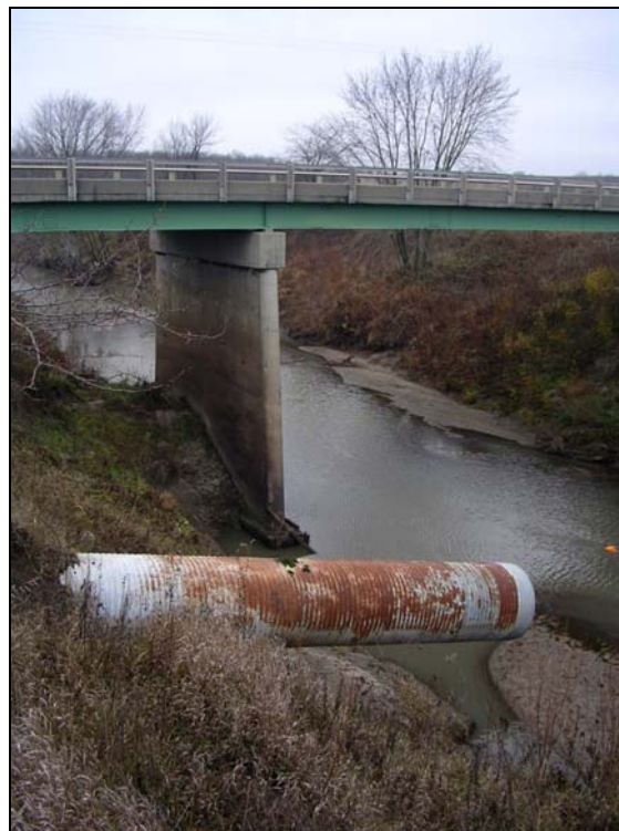
Figure A-10. Improperly designed drainage pipe, aggravating pier scour by contributing to erosion of soil around pier– unknown river in Iowa
