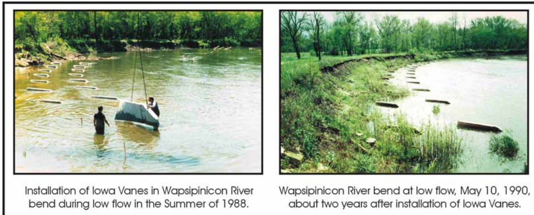
Figure B-22. Vanes installed along the concave bank just upstream from the bridge crossing and their effectiveness in stabilizing eroded bank; Wapsipinicon River in Iowa
