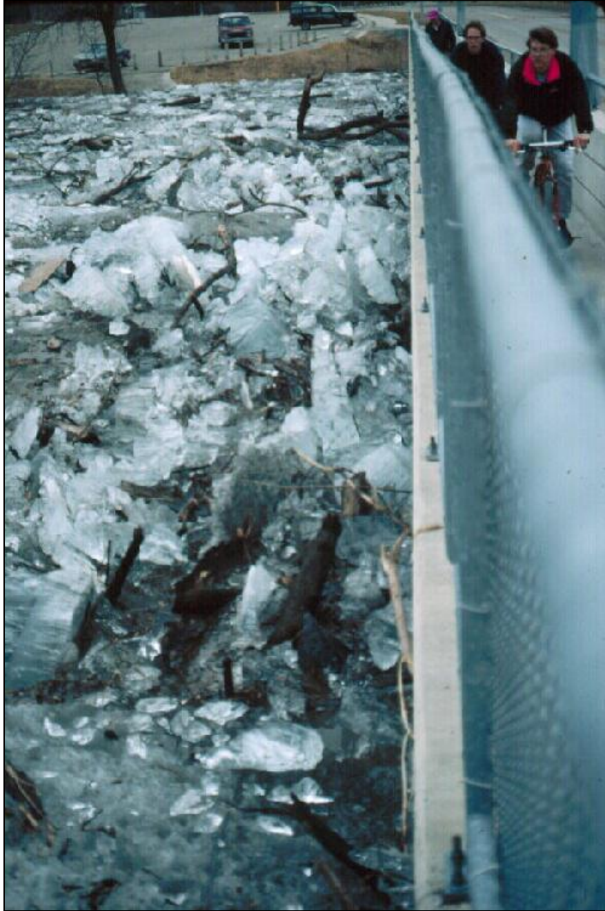
Figure A-40. Ice accumulation along bridge during Spring thaw – Red River, North Dakota
