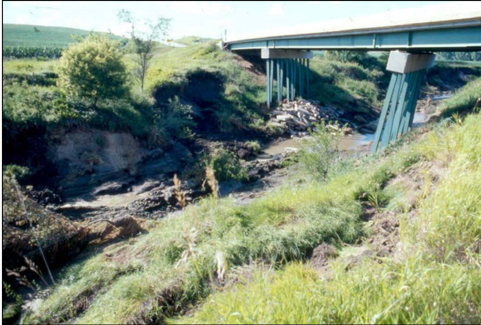
Figure 2-1. Pier failure of a bridge; Willow Creek in western Iowa. The creek had experienced channel degradation (drop in bed elevations) associated with head-cutting (see Chapter 3), which critically reduced support for the pier's piles
