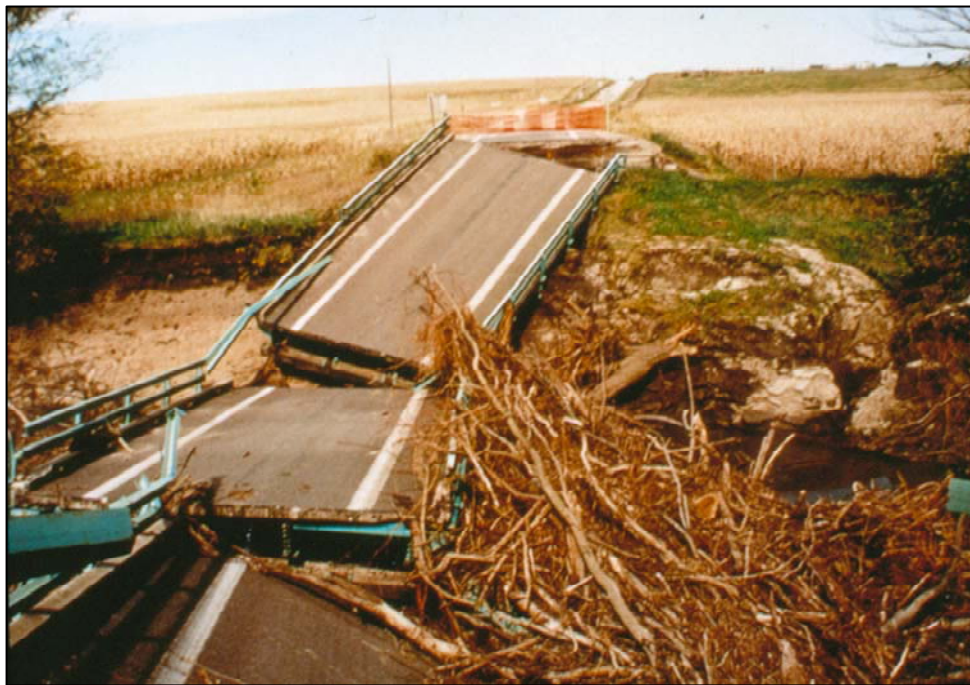
Figure A-37. During flood flow, debris blockage led to high side loads and scour resulting in bridge failure, Florida Creek, Missouri
