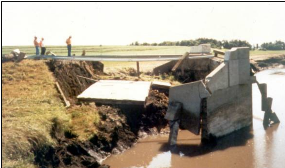
Figure A-30. Washed-out embankment, Brushy Creek, Iowa
