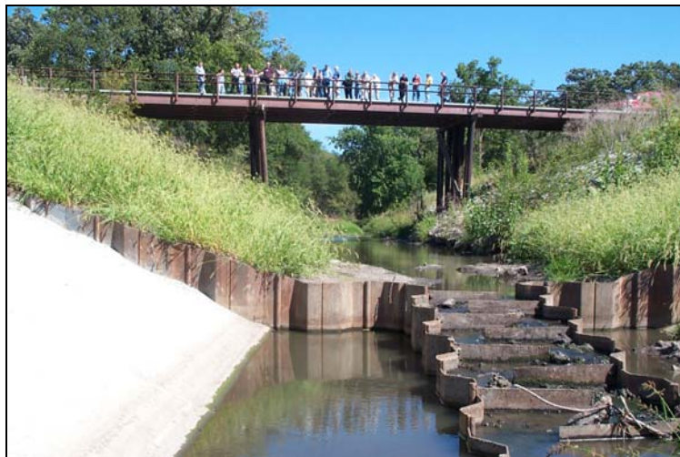
Figure B-35. Combination of sheet-pile weir and fish passage to prevent further stream-bed degradation due to head-cutting, and to enable fish to migrate upstream over the structure, East Tarkio Creek in western Iowa
