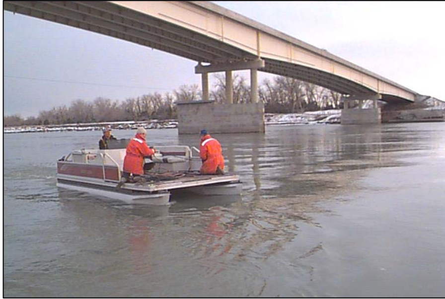
Figure 5-3. Surface-monitoring of bridge waterway conditions by means of boat; Missouri River, Montana
