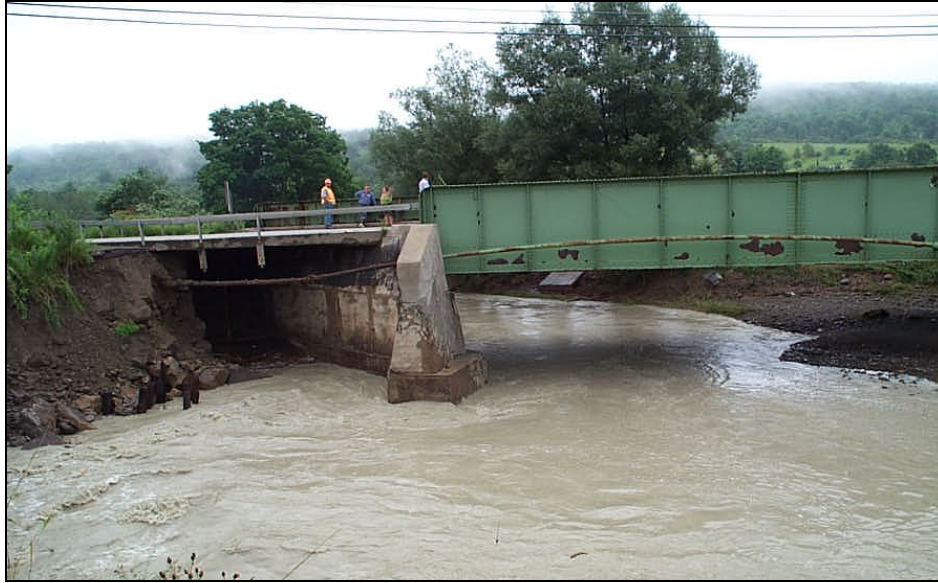
Figure 7-3. Post-flood monitoring of scour at an abutment
