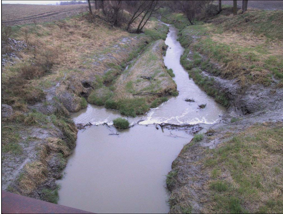
Figure A-42. Downstream channel degradation, Pigeon Creek on L55, Iowa – notice the sheet-pile weir to stop knickpoint migration
