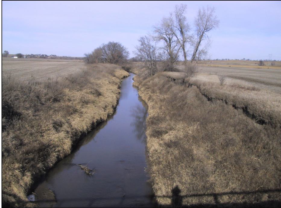
(a) A small straight channel reach - Walnut Creek on gravel road G66 in Pottawattamie County, Iowa (upstream view; notice the bank failure line along the left bank)
