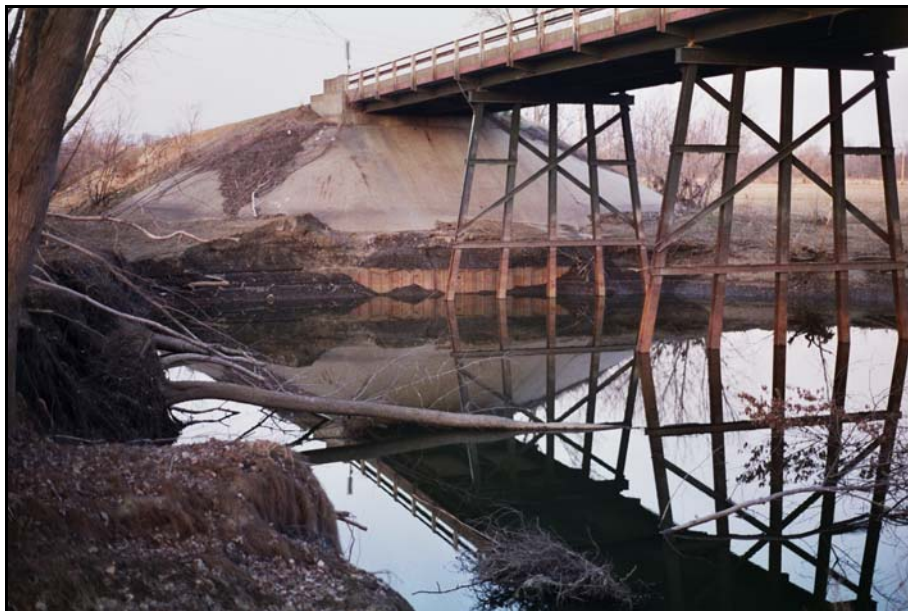
Figure A-32. A large scour hole formed in the floodplain near an abutment and piers of a bridge over the Des Moines River near Chillicothe, Iowa; a substantial amount of flow over the floodplain was forced to pass through the bridge waterway
