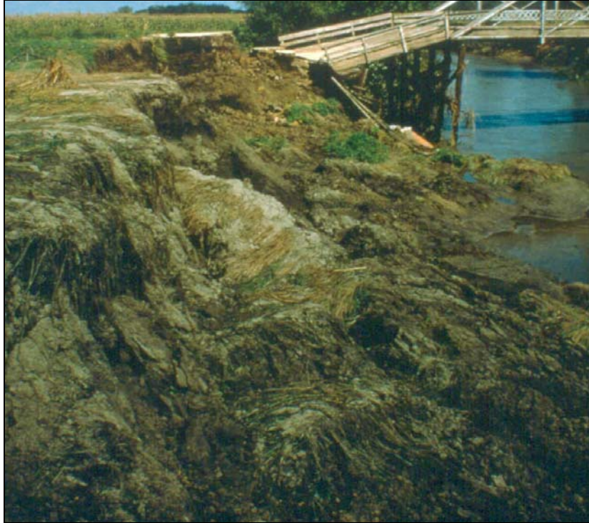
Figure A-4. Failed left bank – unknown river, western Iowa
