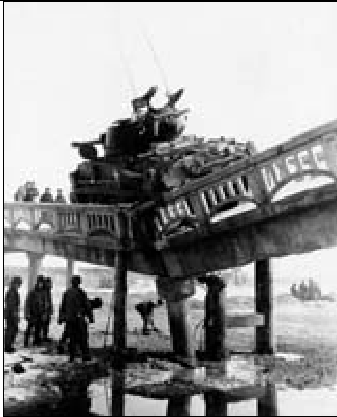
Figure A-15. Pier settlement due to overloading – unknown river
