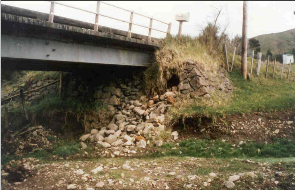
Figure A-22. Local bank failure around abutment – unknown stream, New Zealand
