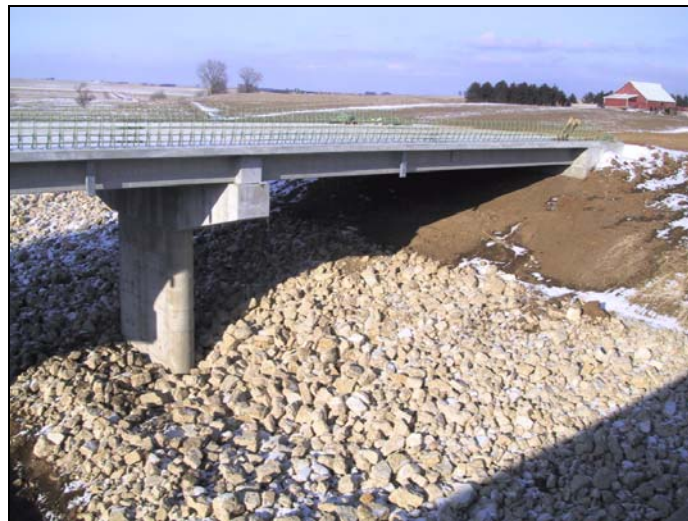
Figure B-2. Heavy riprap protection under construction around piers and abutments Highway 151 bridge; Catfish Creek in Dubuque County, Iowa
