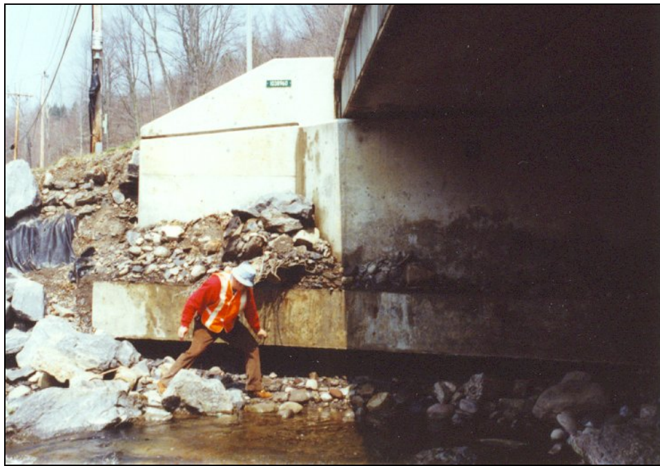
Figure A-26. Inspecting undermined abutment footing, Fulmer Creek, New York
