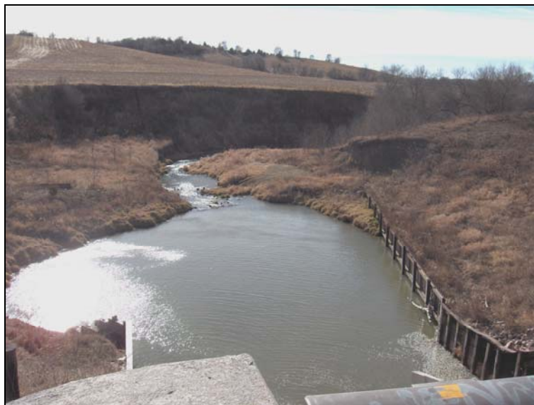
Figure B-37. A downstream view of knickpoint migration that was stopped by a spillway structure -- County Road L16 bridge over Willow Creek, 6 miles upstream of Woodbine, Iowa
