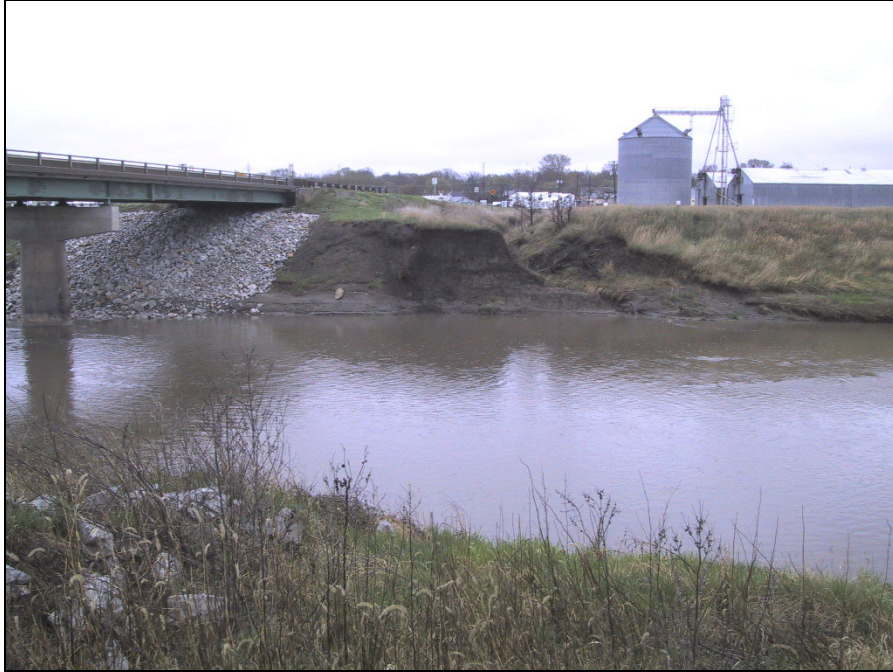
Figure A-31. Partial embankment failure extending from side drainage outlet along the left bank, Boyer River, Iowa
