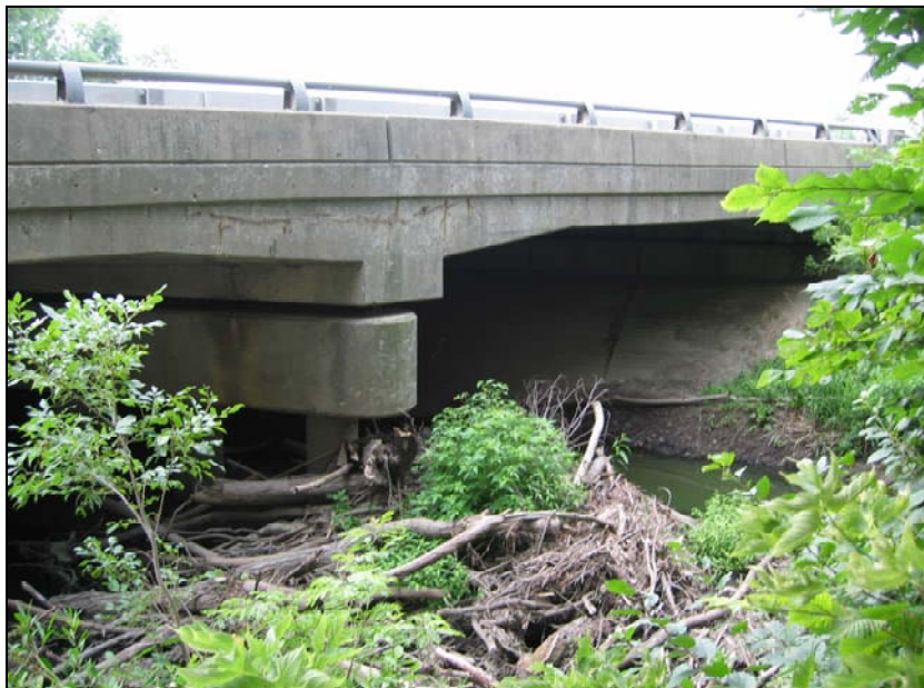
Figure A-35. Vegetation growth on debris at bridge opening, East Skokie Ditch, Illinois
