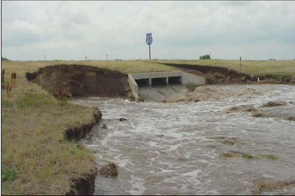
Figure A-46. Scour of embankment at downstream side of culvert; South Platte River, Nebraska
