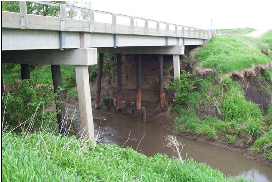
Figure A-11. Pier scour associated with bed degradation (notice initiation of head cutting of side-drainage ditch) – unknown river in Iowa
