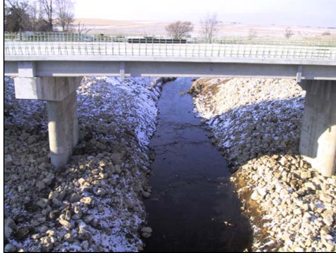
Figure B-1. Heavy riprap protection of low-flow channel and floodplain piers under the bridge on Highway 151 – under construction; Catfish Creek in Dubuque County, Iowa
