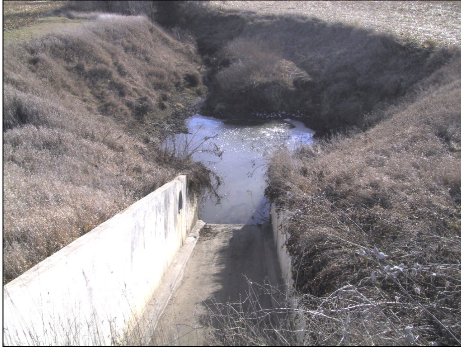
Figure A-48. Large scour hole created downstream from culvert outlet, Walnut Creek on County Road G66, Iowa
