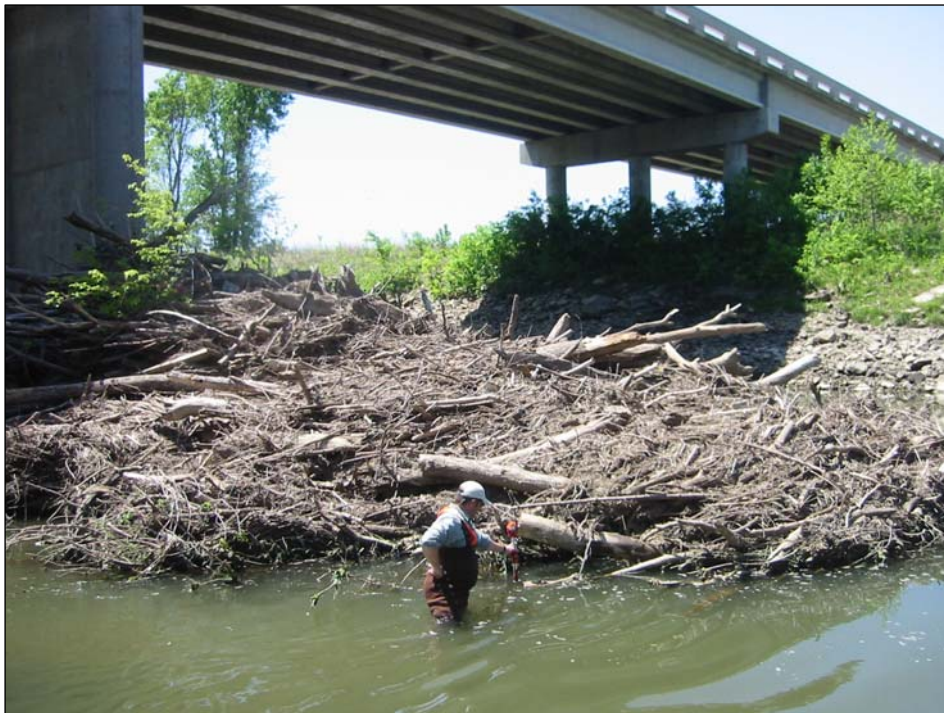
Figure 7-2. Detailed monitoring for scour concerns. In this case, a probing rod is used to measure debris-accumulation thickness at a pier; Verdigris River, Kansas
