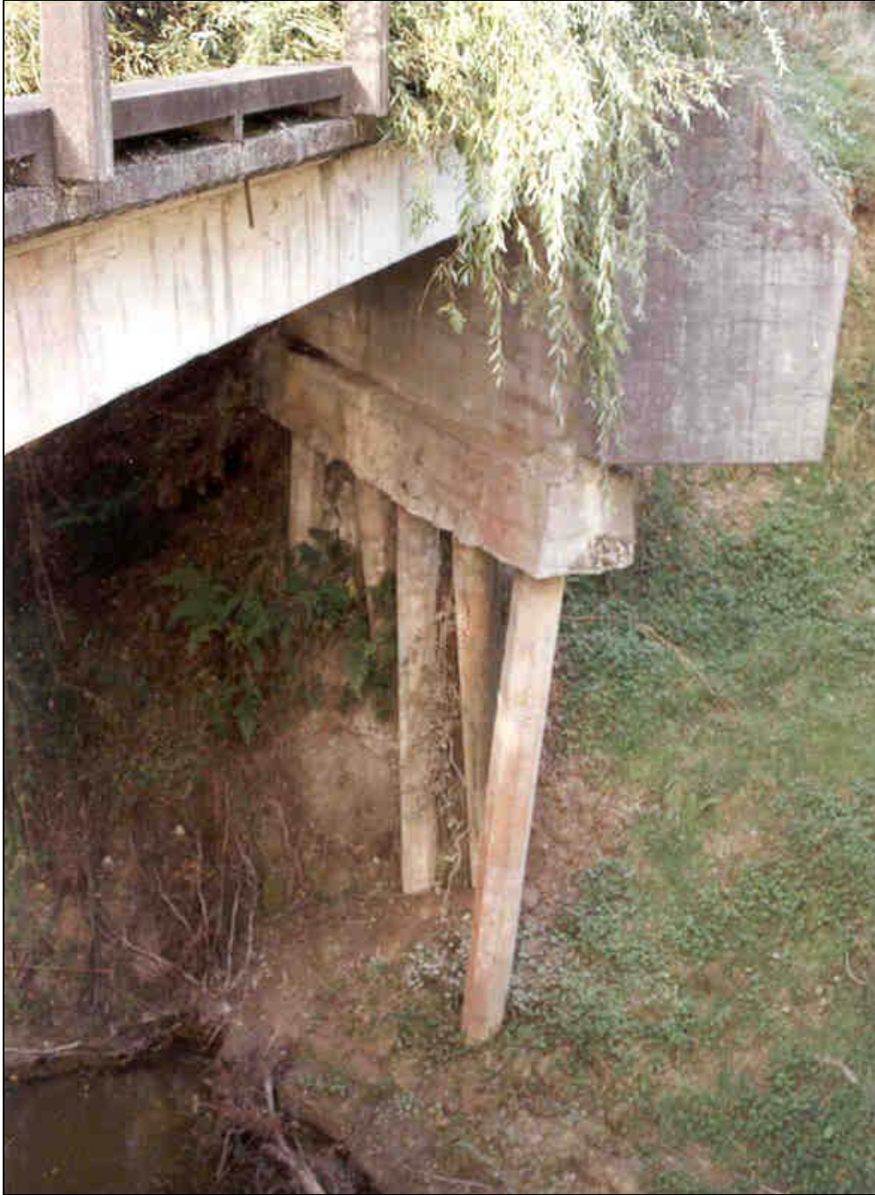
Figure A-24. Abutment scour, unknown river in New Zealand
