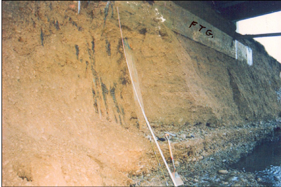
Figure 7-4. Post-flood monitoring of embankment failure at an abutment
