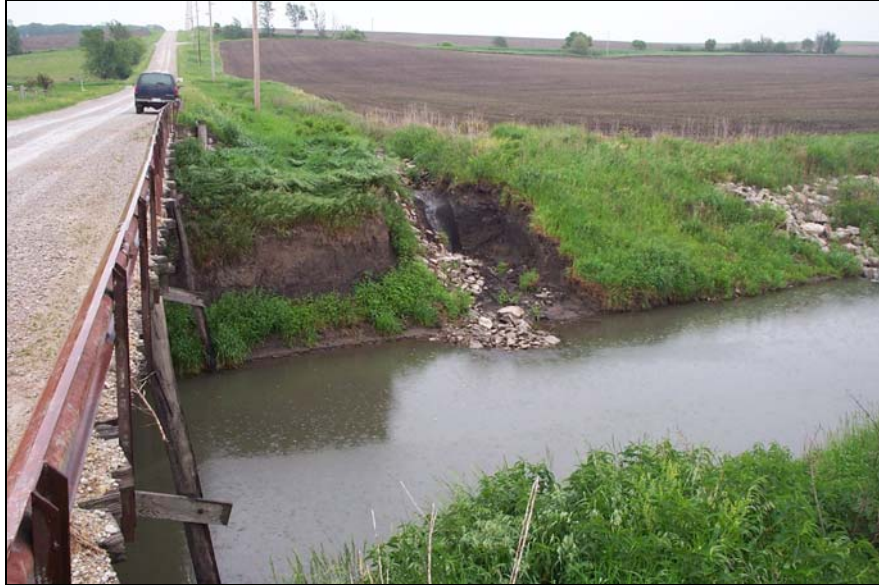
Figure A-9 Head cutting at side drainage upstream from right abutment – unknown river in Iowa
