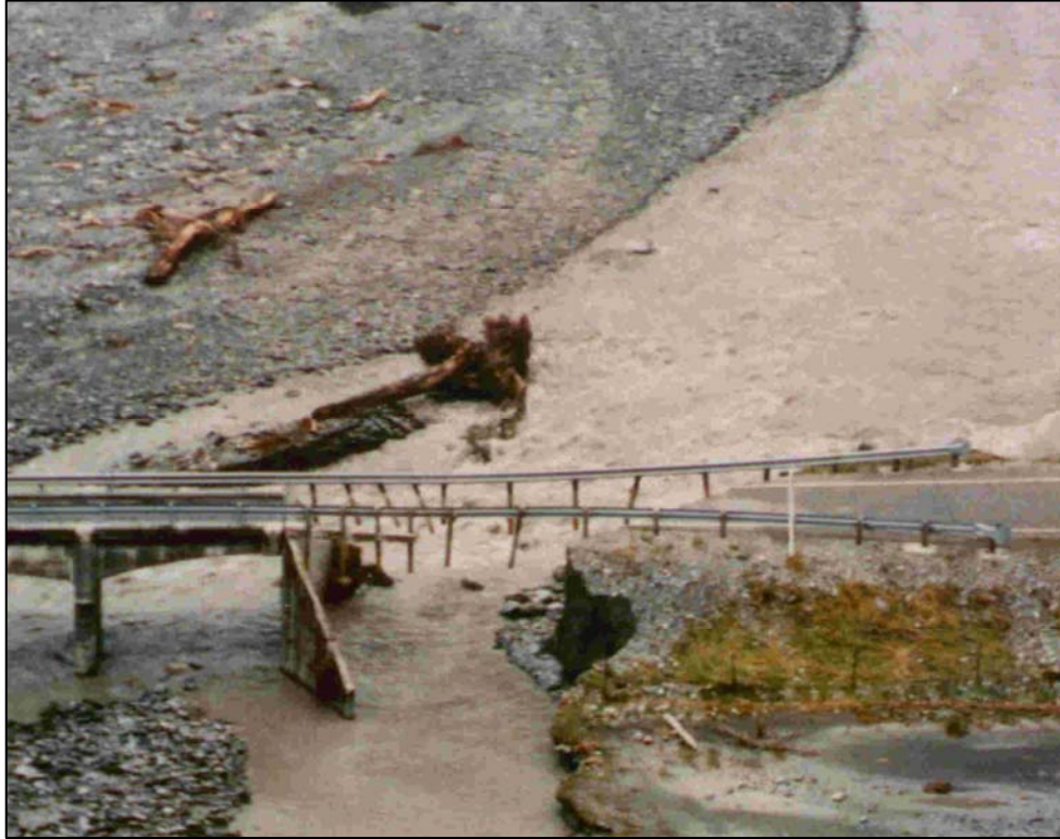
Figure A-29. Failure of embankment and exposure of abutment structure, Camerons Creek, New Zealand
