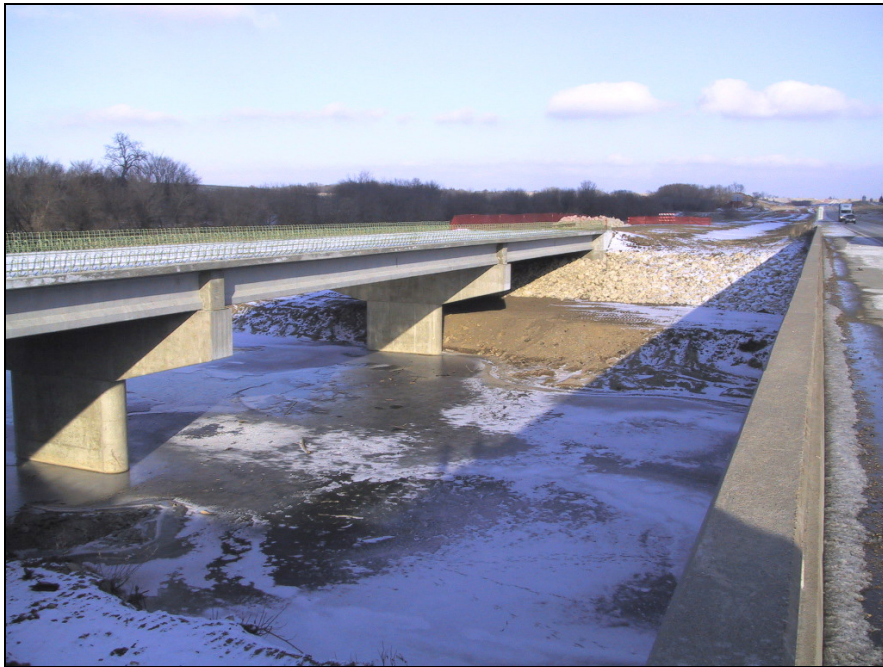
Figure B-6. Abutment protection of the new bridge on Highway 151; Johns Creek in Dubuque County, Iowa
