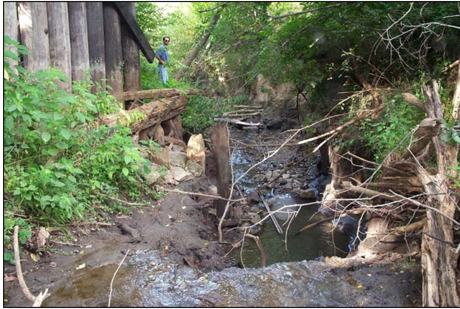
Figure A-44. Headcutting beneath a bridge – Wabash Creek, western Iowa
