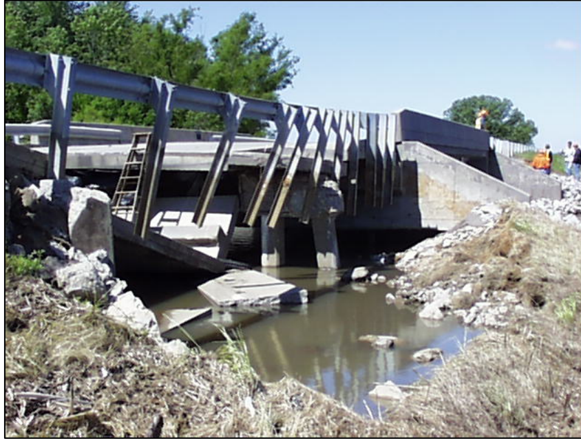
Figure A-34. Washed-out embankment and exposed abutment, I-70 over a small creek, Illinois
