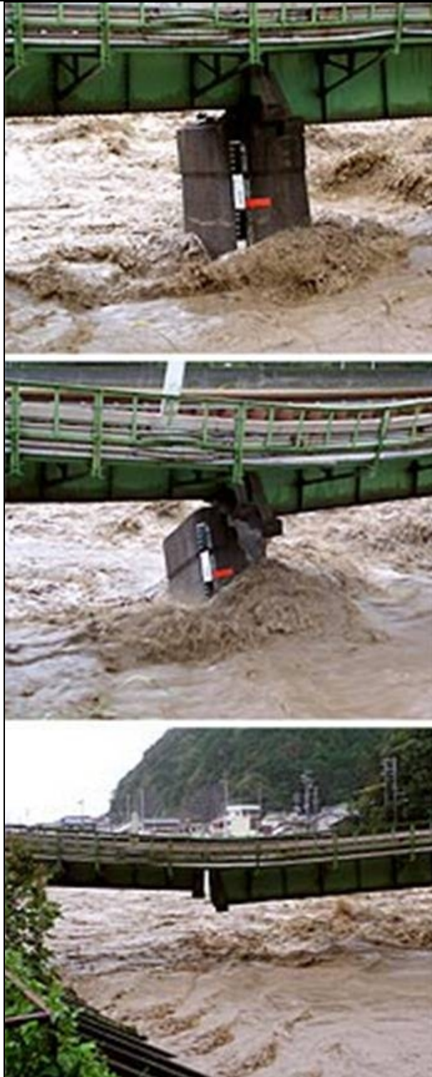
Figure A-19. Pier scour and eventual loss of pier; Akabane River, Japan (courtesy of Prof. T. Hosoda, Kyoto University)
