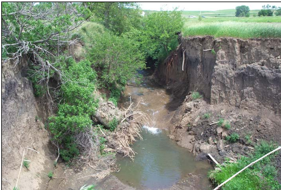
Figure A-43. Headcutting; unknown stream in Iowa
