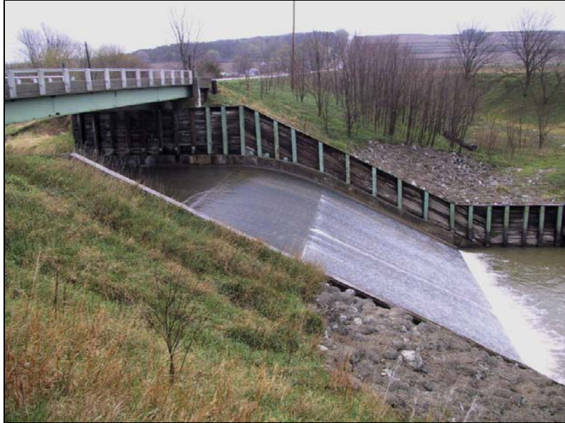
Figure B-38. A concrete spillway constructed to stop knickpoint migration, Willow Creek in Harrison County, Iowa. The weir and bridge abutments form what in Iowa is known as a "Greenwood Bridge"
