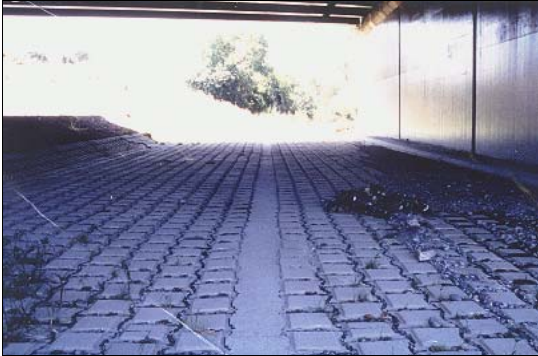
Figure B-32. A further example of the use of cable-tied blocks for scour protection between abutment and first pier
