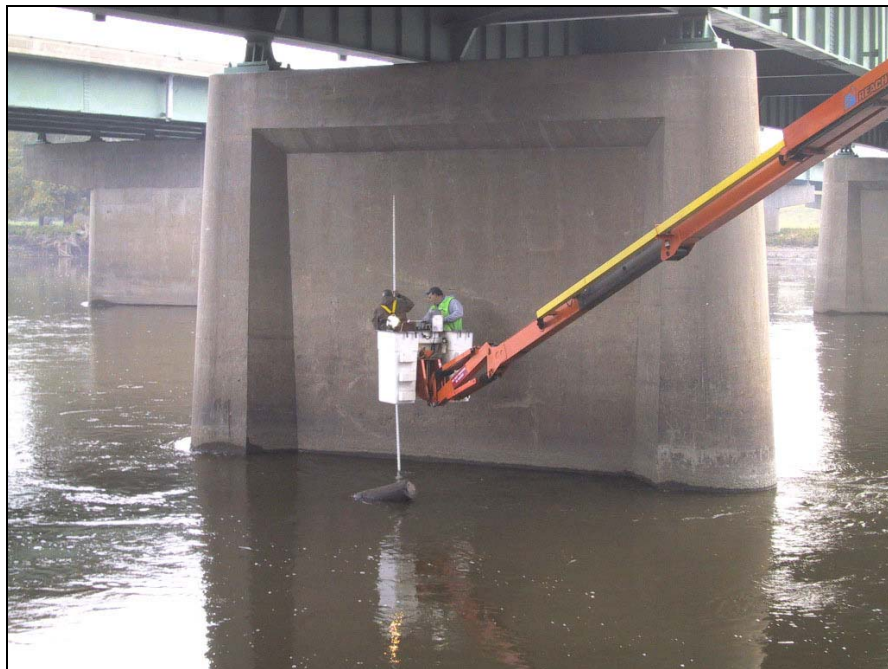
Figure 5-2. Access by means of a truck-mounted telescopic boom. Equipment of this scale usually is used by the Iowa DOT, Highway 151 bridge over Cedar River, Iowa
