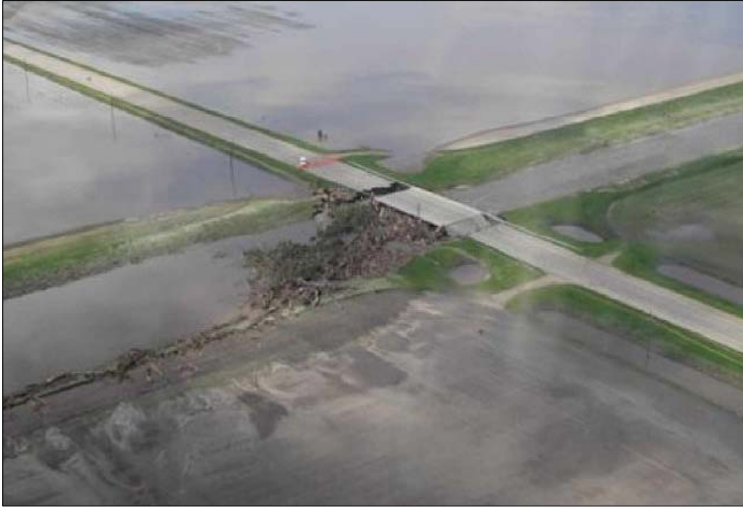
Figure 1-4. Debris accumulation at a small bridge results in abutment scour and flooding; Wild Rice River, Minnesota
