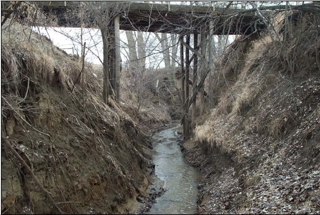
Figure A-41. Channel degradation owing to knickpoint migration – unknown river in western Iowa
