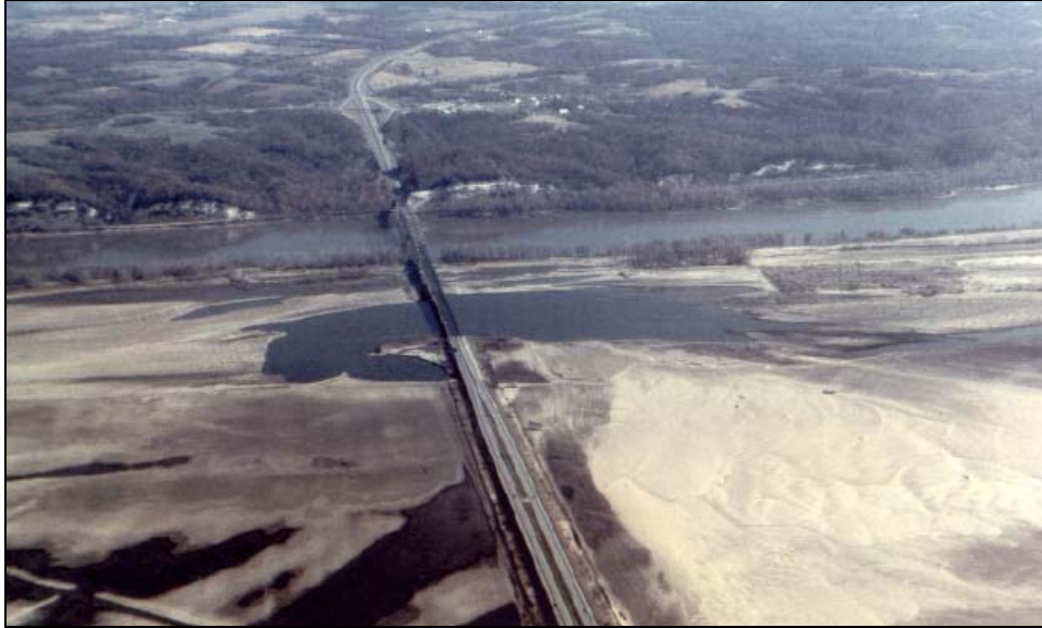
Figure A-27. Scour at abutment on floodplain of Missouri River, I-70, Kansas
