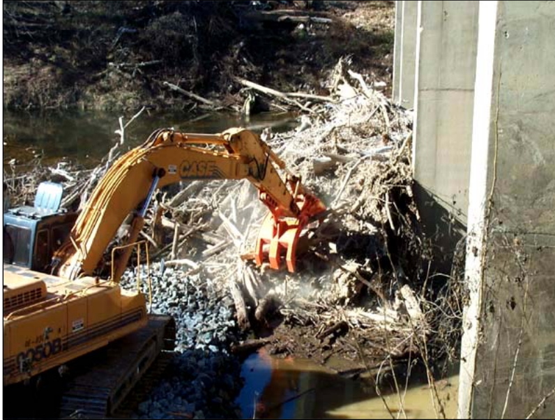
Figure B-13. Removal of woody debris by a backhoe grab; Deep River, North Carolina
