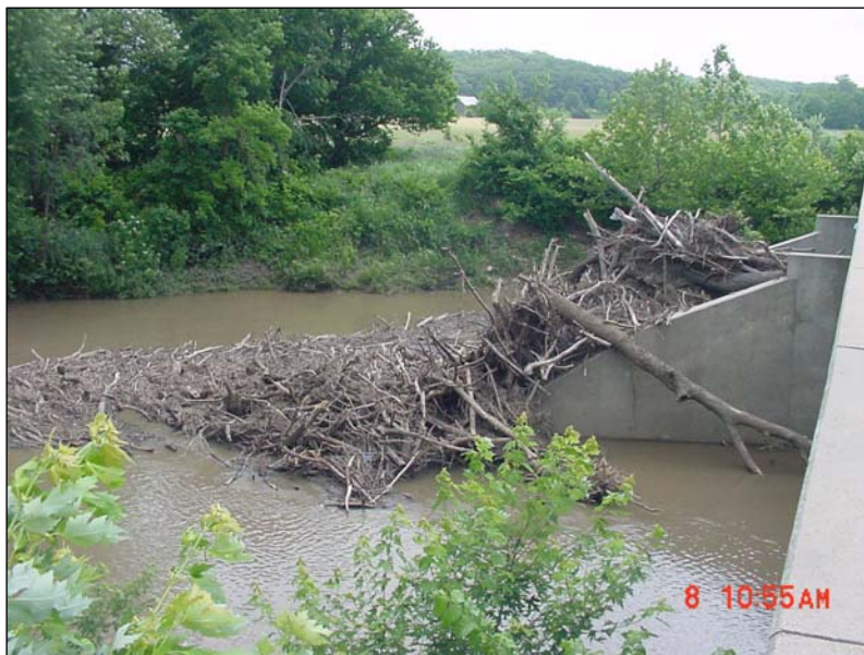
Figure B-10. Pier-nose walls added to a bridge in order to fend debris from the bridge deck; Elk River, Kansas
