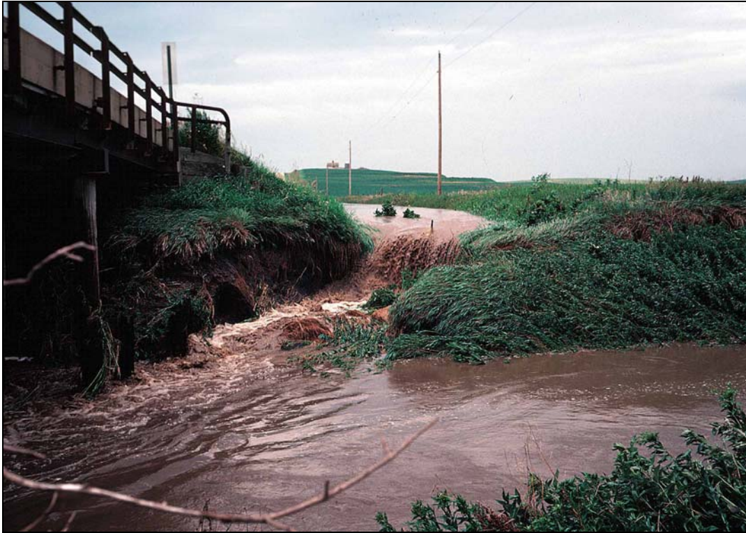
Figure A-8. Flow from side drainage ditch eroding the right bank – unknown river in Iowa
