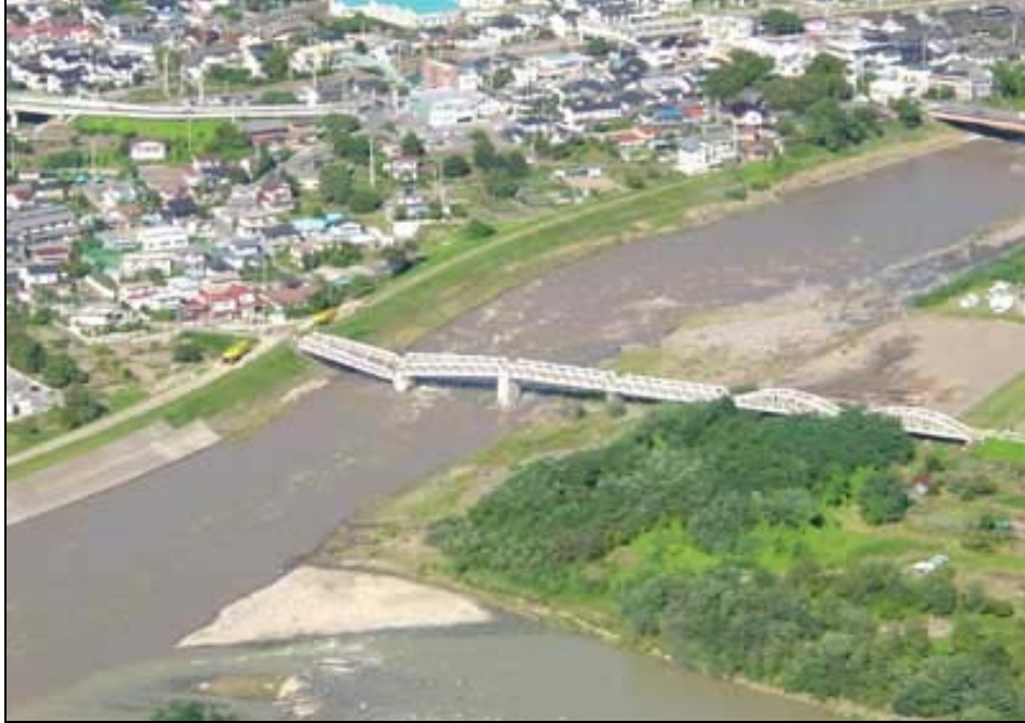
Figure A-17. Pier scour, Chikuma River, Japan (courtesy of Prof. T. Hosoda, Kyoto University)
