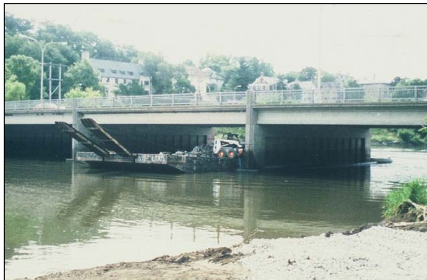
Figure B-4 Placing rock riprap as a mound around exposed pile supports of a bridge pier in a channel that has experienced general bed degradation; Iowa River in Iowa City, Iowa, below Coralville Reservoir
