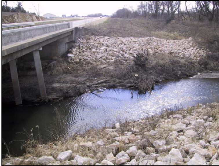
Figure B-34. Downstream bank protection of Highway 151 bridge, Kitty Creek in western Iowa
