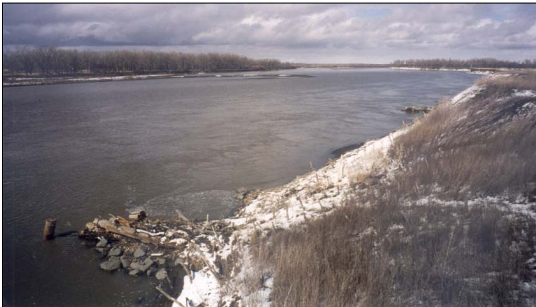
Figure B-26. Timber hard points reinforced by riprap along the concave bank; Missouri River, Montana
