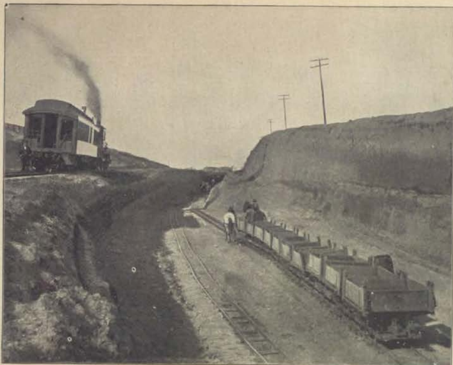
CHICAGO GREAT WESTERN RAILWAY. View showing the character of work in progress in Iowa where ruling grades are being reduced.
