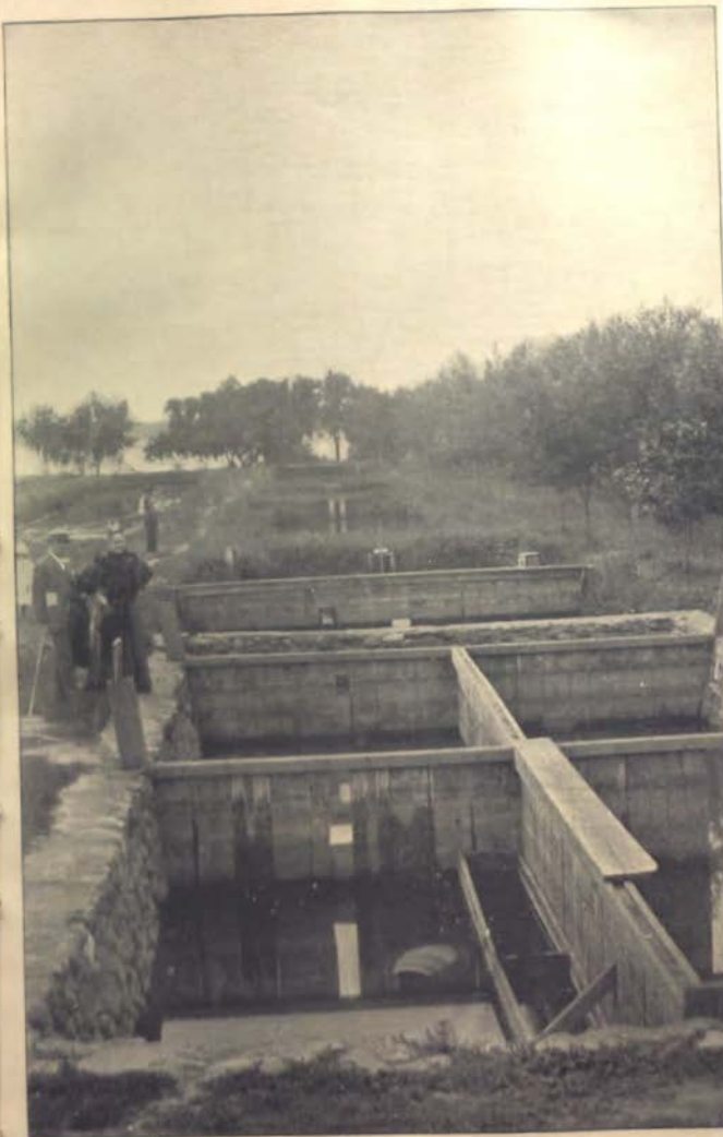
Hatching Ponds, State Hatchery.
