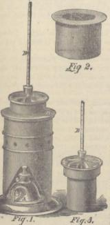
Fig. 1 represents the instrument entire. It consists of a sheet copper stand 8½ inches high, exclusive of the base, and 4½ inches in diameter. On one side is an aperture 3½ inches high for introducing a small spirit lamp. **A**, or better a small gas-burner, instead of a lamp, when gas is available.
