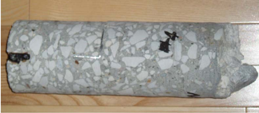
Figure G4. Test section 4 core
