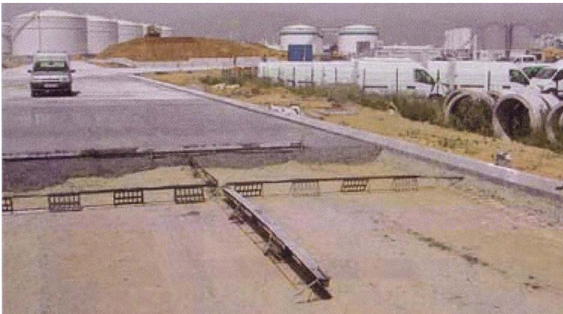
Figure 1. JRI+ joint before concrete placement
