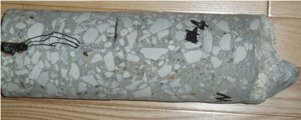
Figure G5. Crack in test section 4 core
