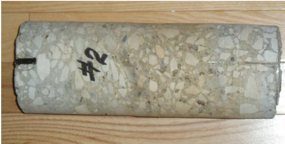
Figure G2. Test section 2 core
