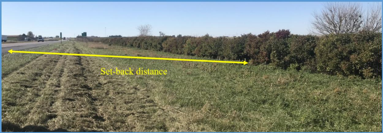
Figure 8. Living fence locates on I-35, Iowa. The set-back from right of way is 18 meters (59 feet).
